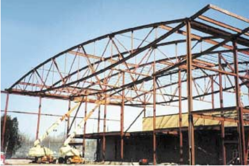
Side view close-up of double-bowed Oneida Junior/Senior High School gymnasium truss
