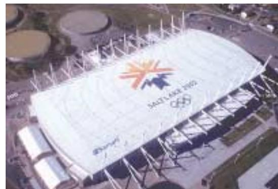
atically lowered roof ...makes it cheaper to heat and cool the arena." The smaller enclosed volume also allows for optimum indoor air temperatures for skating and for ice control.
