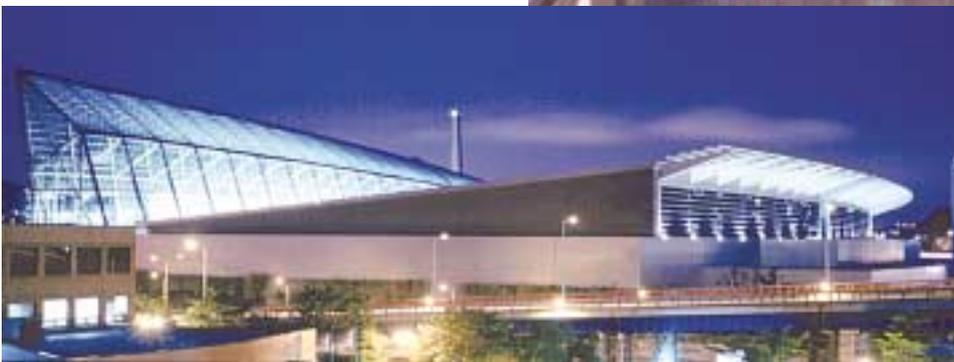
**A** progressive harbor city poised on the Sea of Japan, Pusan, Korea, is now the home to a convention center and exhibition hall composed of a prismatic glass gallery and a dramatically sloped roof. Both building elements are structured in steel in this 900,000 sq. ft. flagship convention and exhibition facility.
