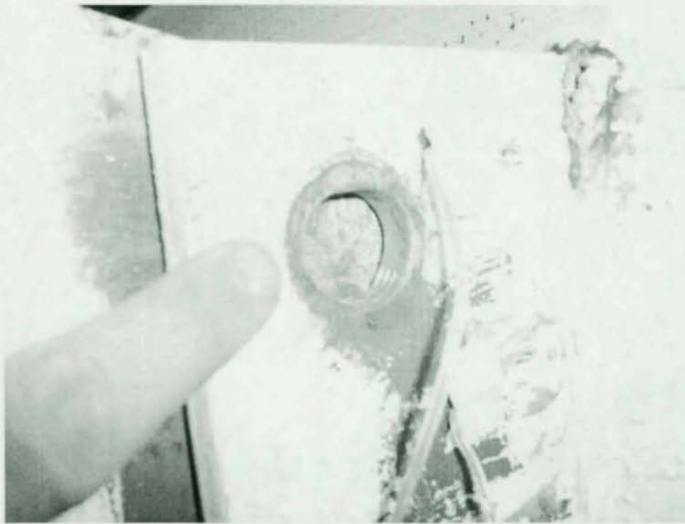
Test 7A – Top Bolt Hole in Shear Tab at End of Test
