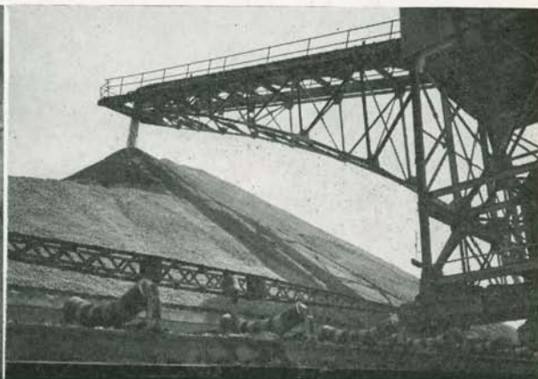
Traveling conveying stacker at The Inland Lime & Stone Company plant.
