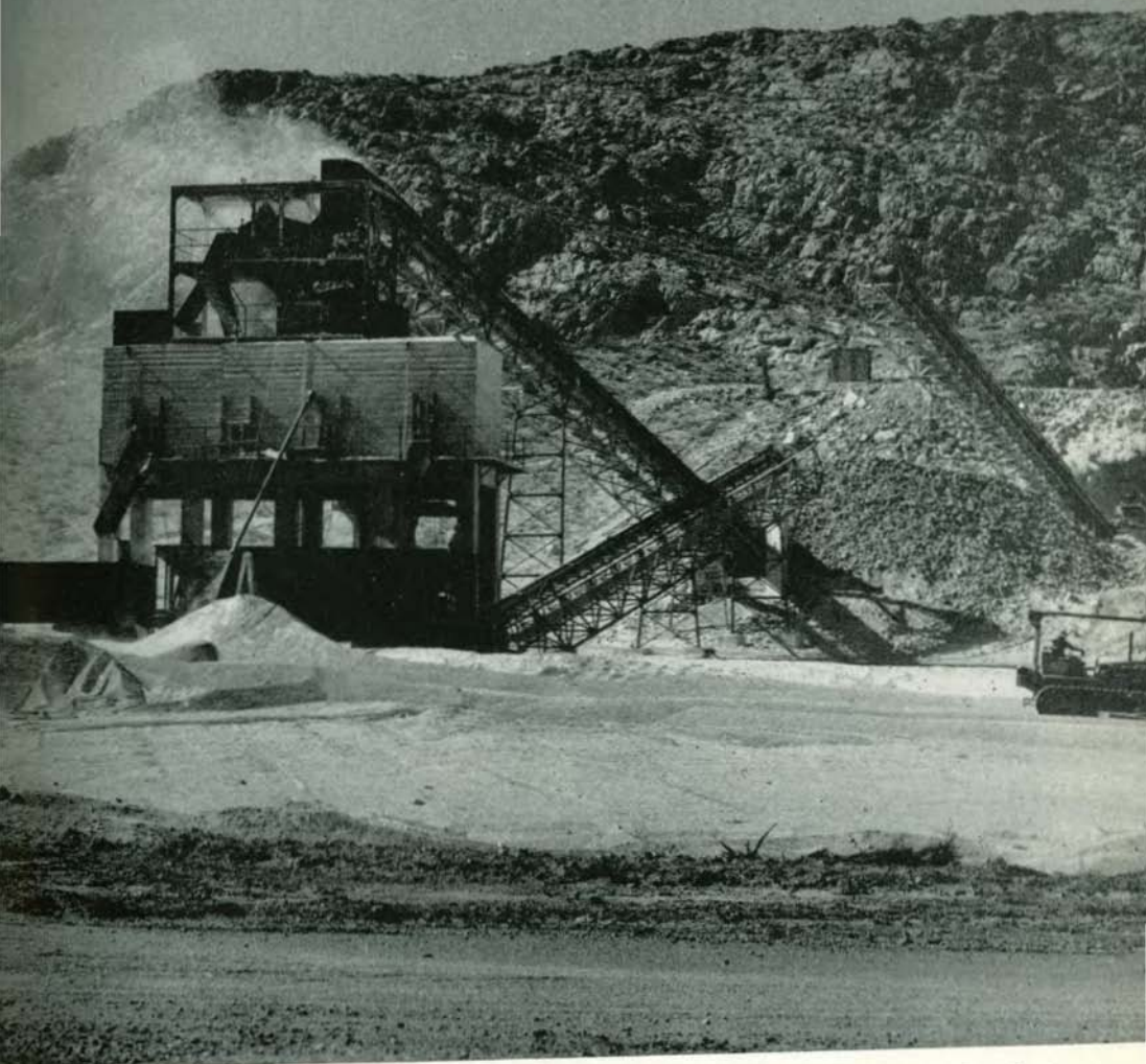
Besides iron ore and coal, the third raw material needed for Fontana's pig iron producing blast furnaces is limestone, which is supplied from Nevada deposits.
