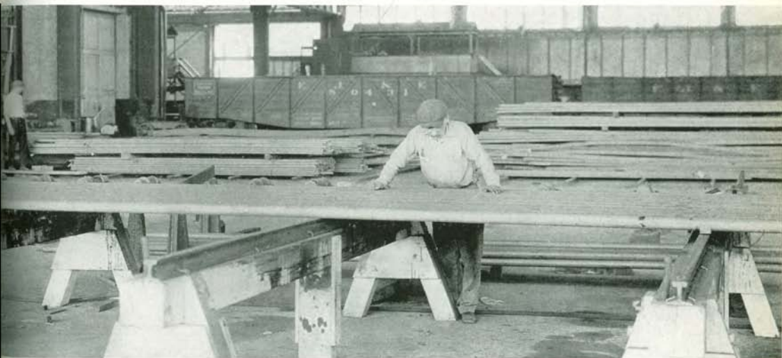
A trained workman is examining 3½% nickel alloy 3" rounds for possible surface defects
