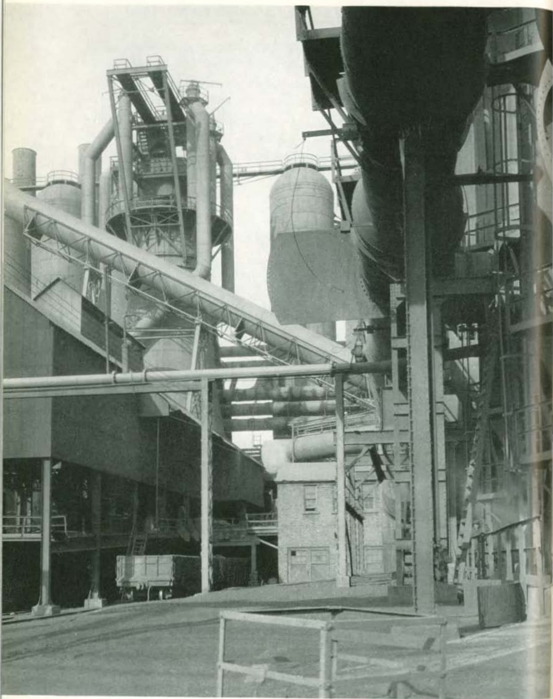
A close-up of a blast furnace in which ore, limestone and coke are heated to produce molten iron
