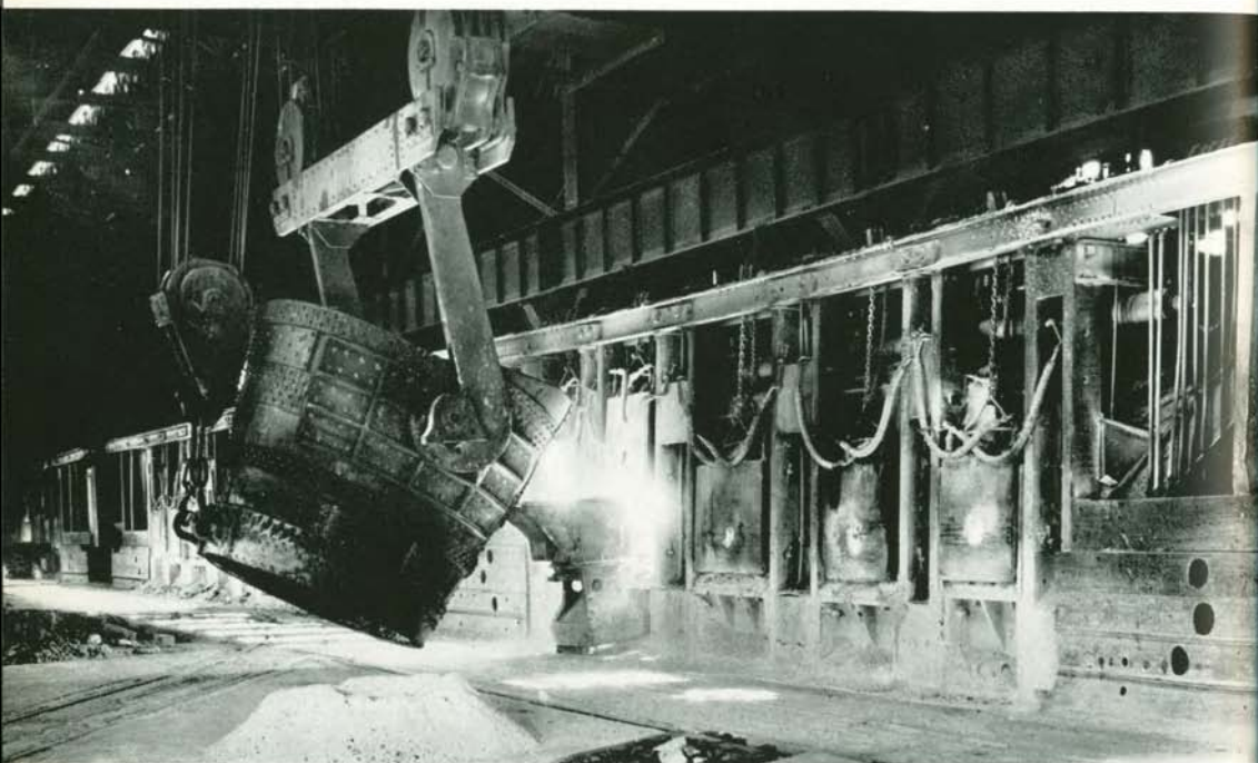
This giant bucket is charging an open hearth furnace with molten metal from the blast furnace
