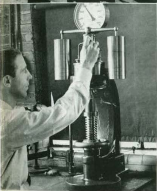
Making a Brinell hardness test
