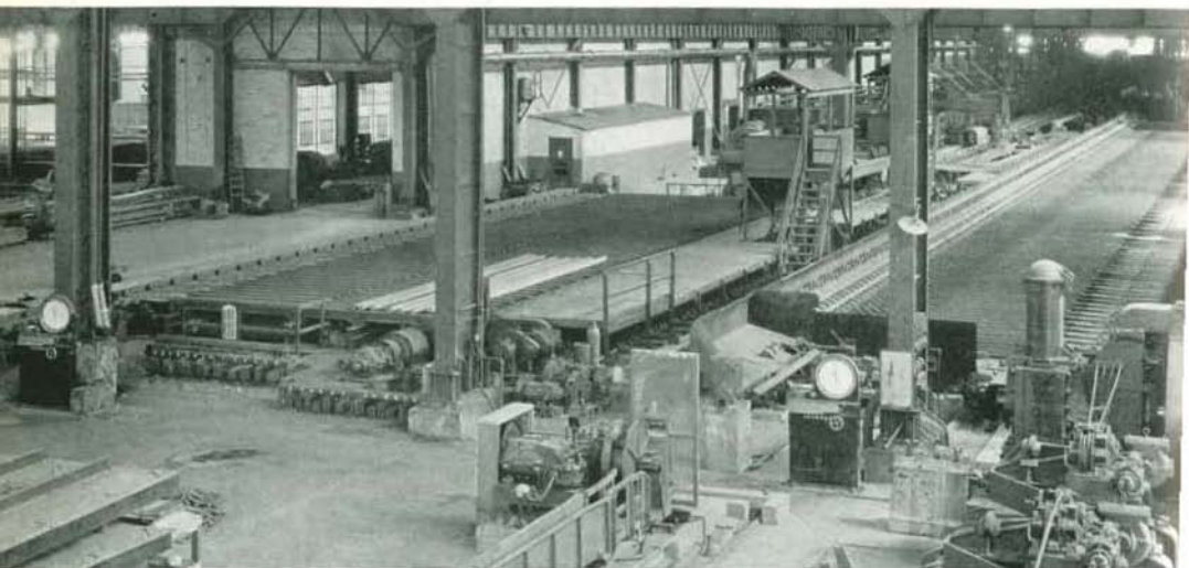
In this section of the mill alloy bars are accurately sheared to length
