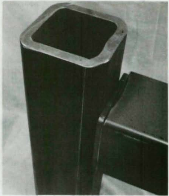
CJP with backing (Key 5). TS 4x4x1/8" onto TS 4x4x \frac{1}{2} ".
