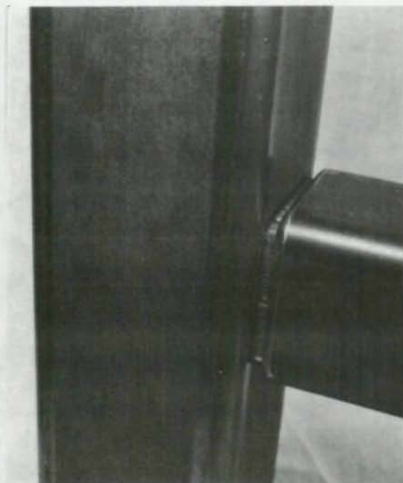
CJP with backing (Key 9).
