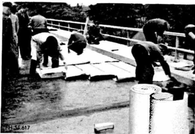
Fig. 8.3. Rippled aluminum foil sheets being placed on a steel plate deck. Bonding compound used for adhesion to steel
