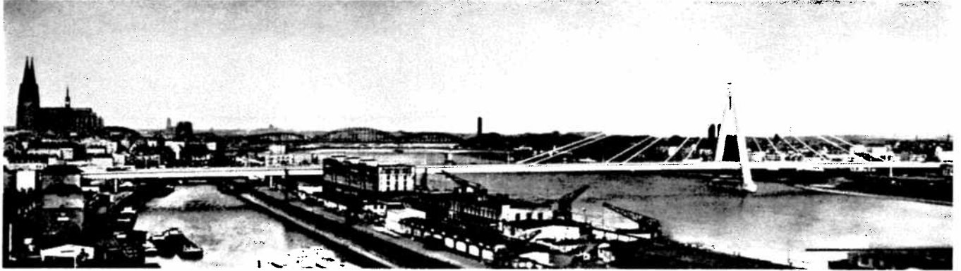
Fig. 1.18. General view of Severin Bridge, Cologne
