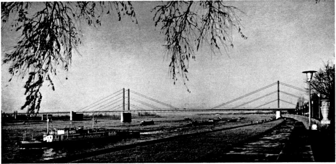
Fig. 1.16. View of Duesseldorf-North Bridge
