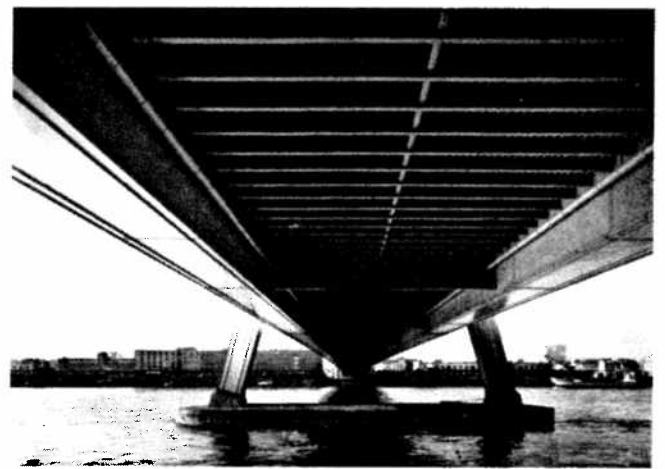
Fig. 1.20. Underside view of Severin Bridge
