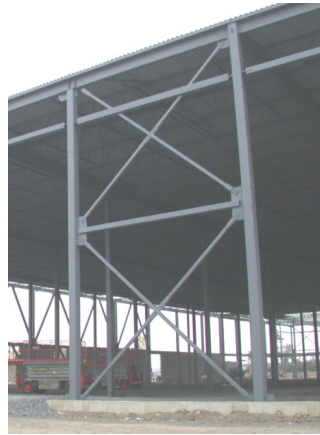
Figure 1. Two-tier concentrically braced frame (Imanpour and Tremblay 2012).
