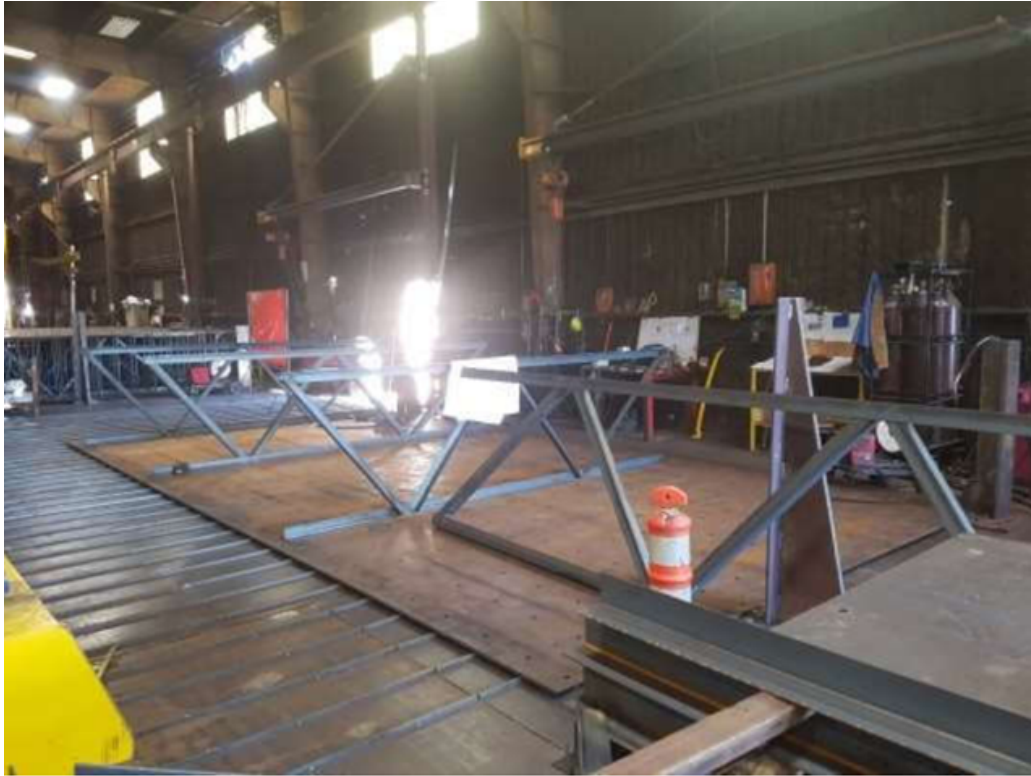
Figure 20: Panel Stabilizing Frames Being Fitup on SpeedCore Wall Module
