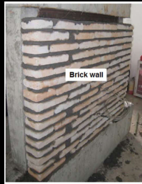
Brick wall on unexposed surface
