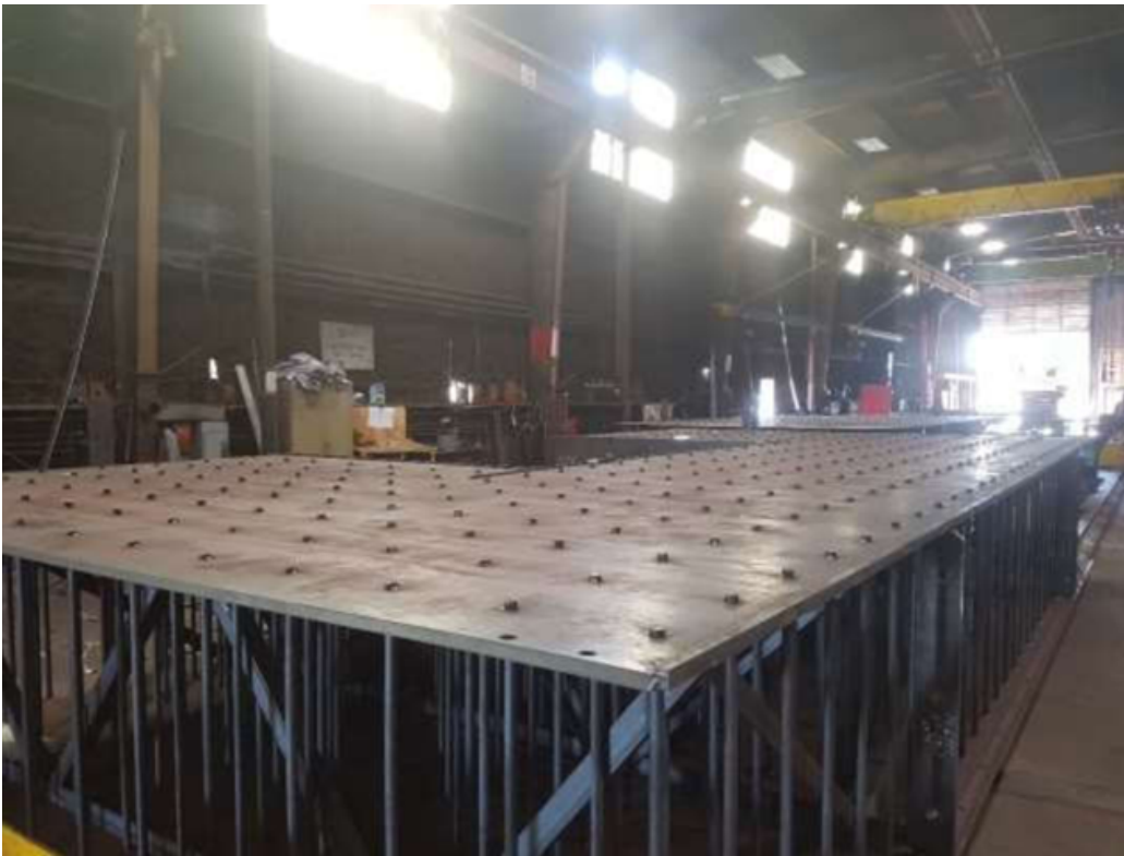
Figure 21: Fully Assembled Wall Module Showing Installed Stabilizing Frames
