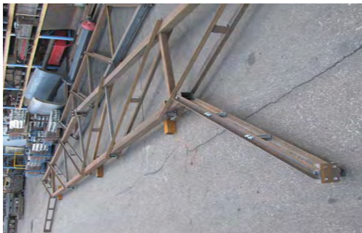
Figure 10. Inner frame after assembly.
