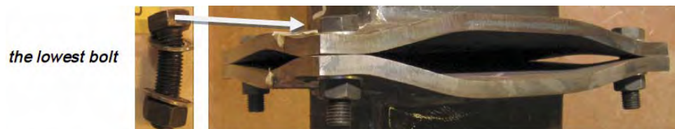
Figure 6. Deformations after test TE2 ( t_{pn}=15 mm), slight necking of the bolt.
