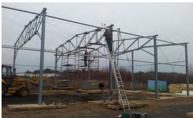
Figure 11. Testing truss frame of industrial hall
