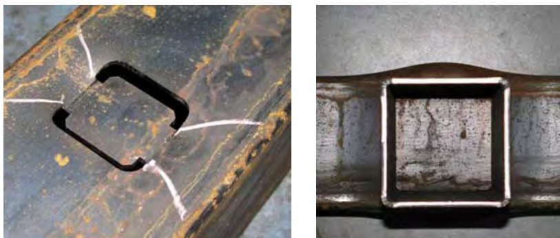
Figure 3. Chord upper wall failure (WTL1) & chord side walls failure (WTL3).
