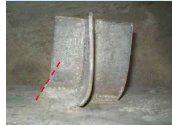
Figure 2. Cross type shear lug
