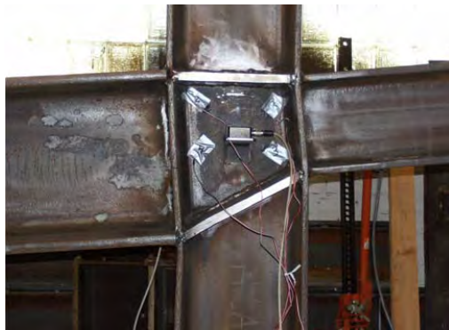
Figure 9a. Panel inelastic deformation
