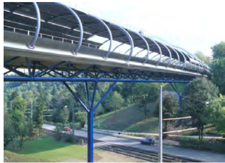
Figure 4. Nesenbach Bridge (Puthli et al. 2010)
