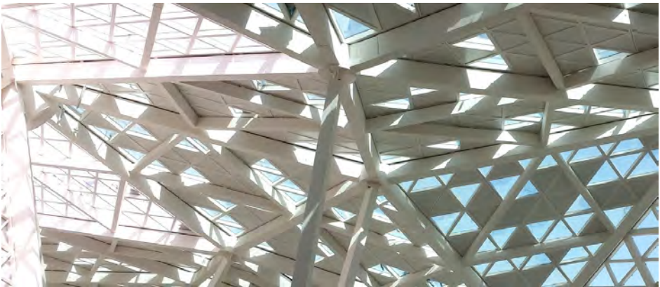
Figure 16: The completed Structure
