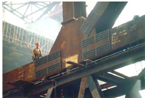
Figure 5: Transfer Truss Bottom Chord
