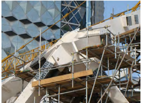
Figure 15: Connecting members to node
