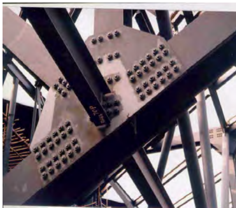
Figure 6: Long Span Truss Bottom Chord
