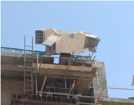
Figure 14: Node being positioned on site
