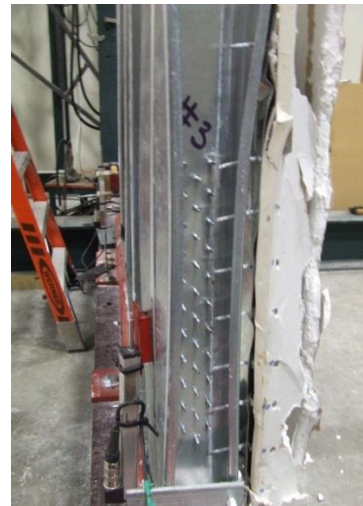
Figure 7: Screw pull out failure
