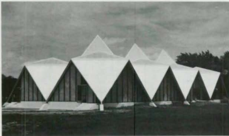
After the structural steel frame was in place (above), the three high pyramids were covered with triangular sections of translucent white plastic and the remainder of the structure was sheathed in corrugated aluminum (below). The interior beams were painted boat-blue and left exposed.
