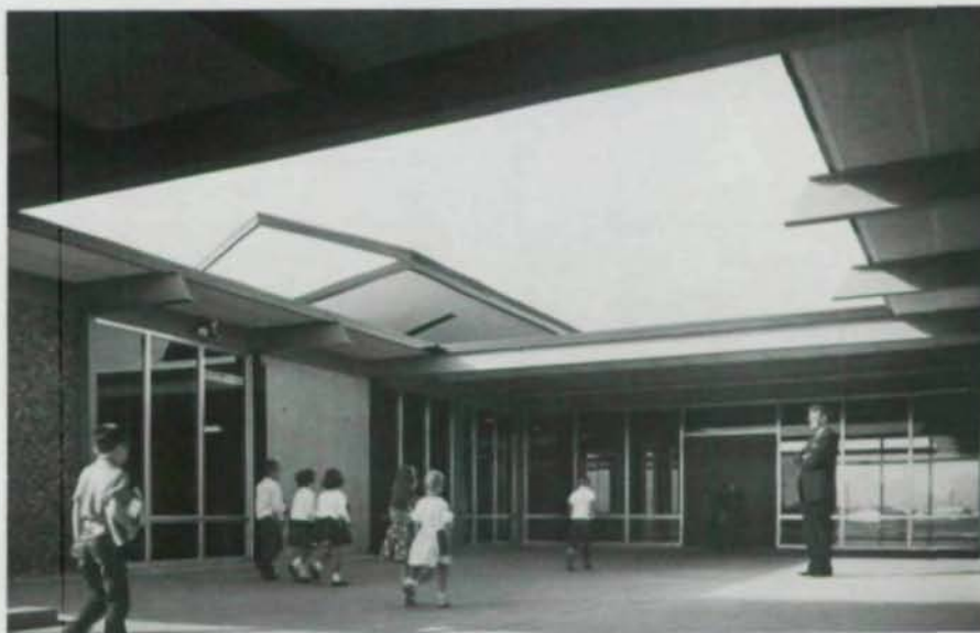
Floor plan (above) demonstrates how architects solved the problem of access from any classroom to the rest of the building as well as egress from each room to the outdoors. Interior court (below) shows detailing of the structural steel as well as exterior panels of exposed aggregate finish. Panels were cast at the site, then lifted and bolted to the steel frame.
