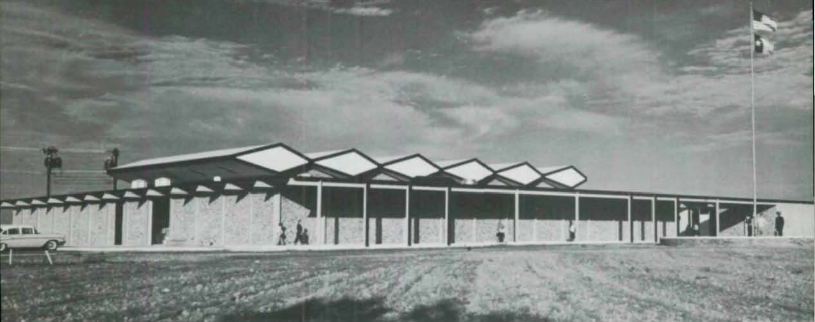
Front facade of the Abilene, Texas. Elementary School shows the unusual diamond trusses over the cafetorium.
