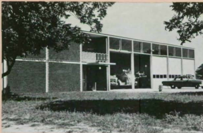
Bethany Fire Station Bethany, Okla. Architect: Locke, Miner & Smith, Inc.
