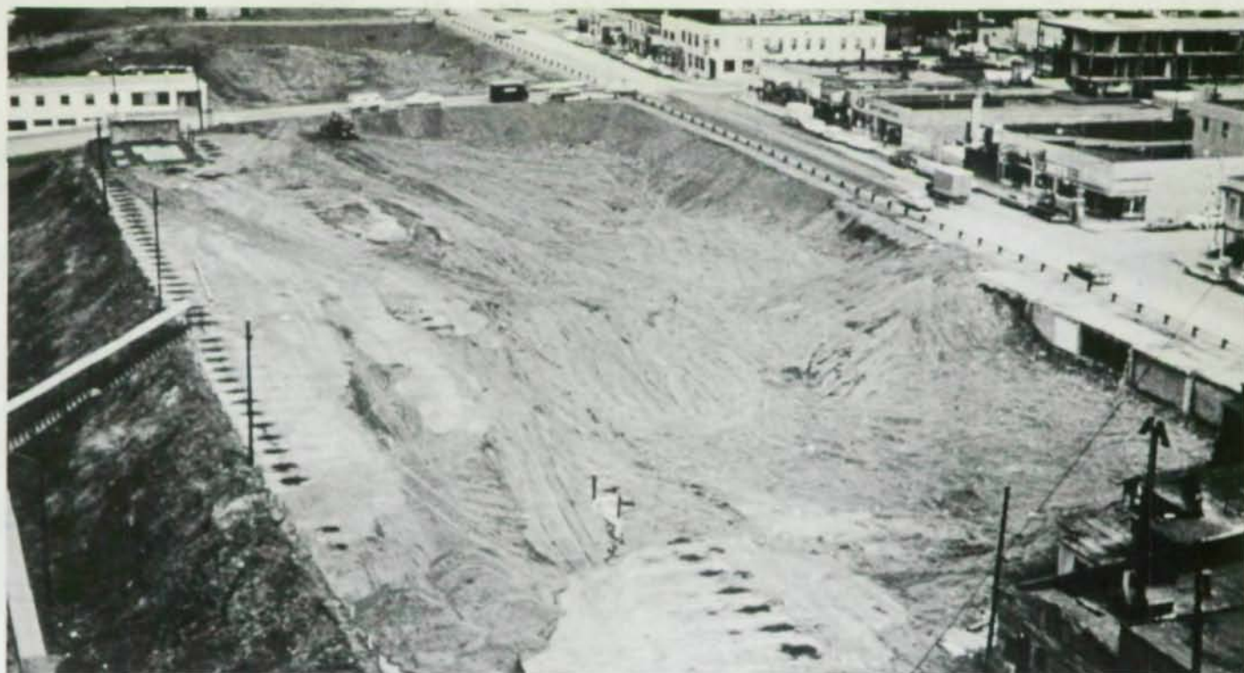
Fourth Avenue from top of Westward Hotel
