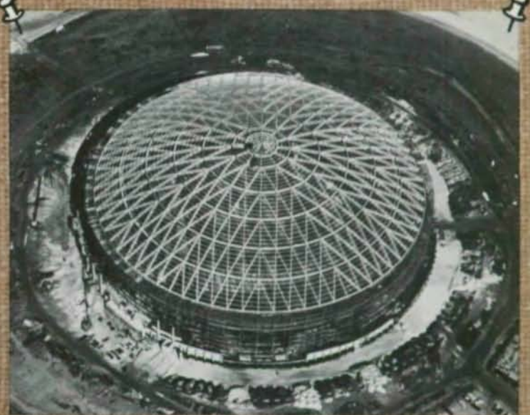
Harris County Domed Stadium, Houston, Texas
