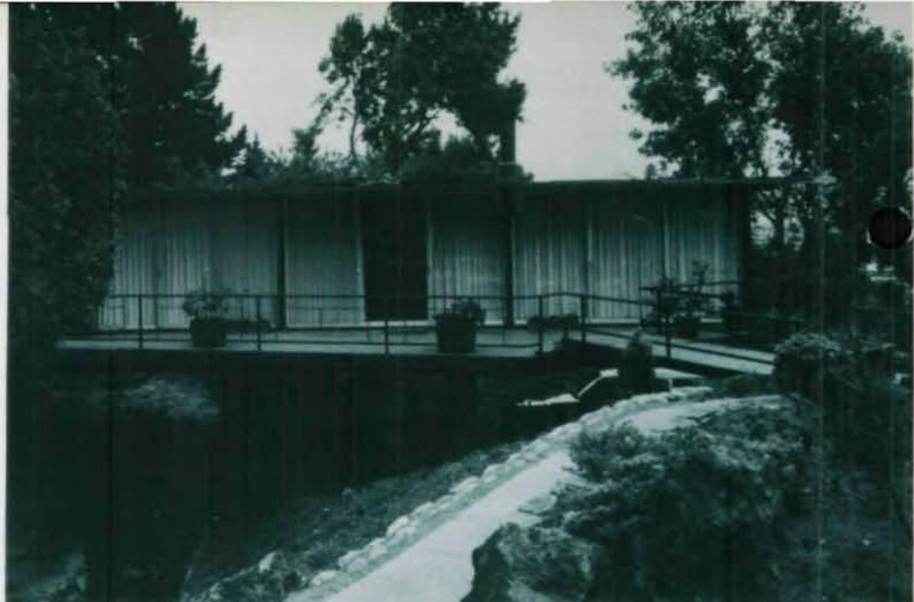
Entire house is framed in steel, much of it exposed and painted black. A footbridge, hand-railings, spiral stairway, and fireplace — all of steel — complement the structural skeleton.
