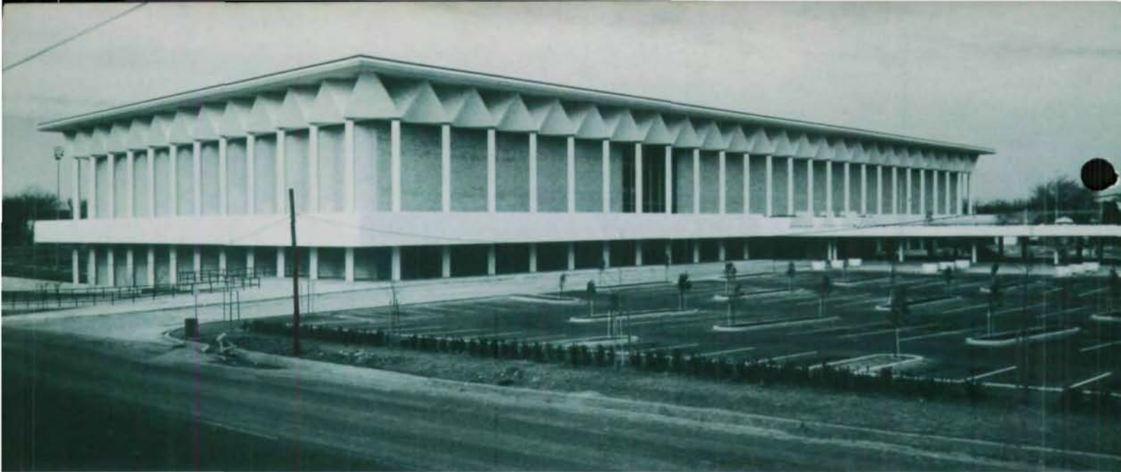
STEEL REPLACED CONCRETE IN ORIGINAL DESIGN. EDWARD DURELL STONE WAS ARCHITECT, WITH MURRAY-JONES-MURRAY AS ASSOCIATES.
