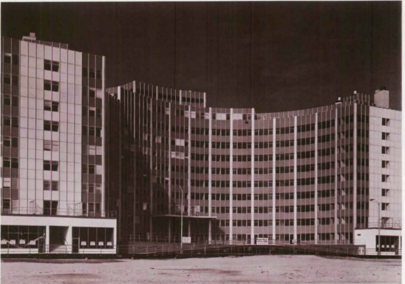
Steel framing saved 12.5% in construction of $4.5-million Ocean Manor Apartments on Atlantic City boardwalks.
