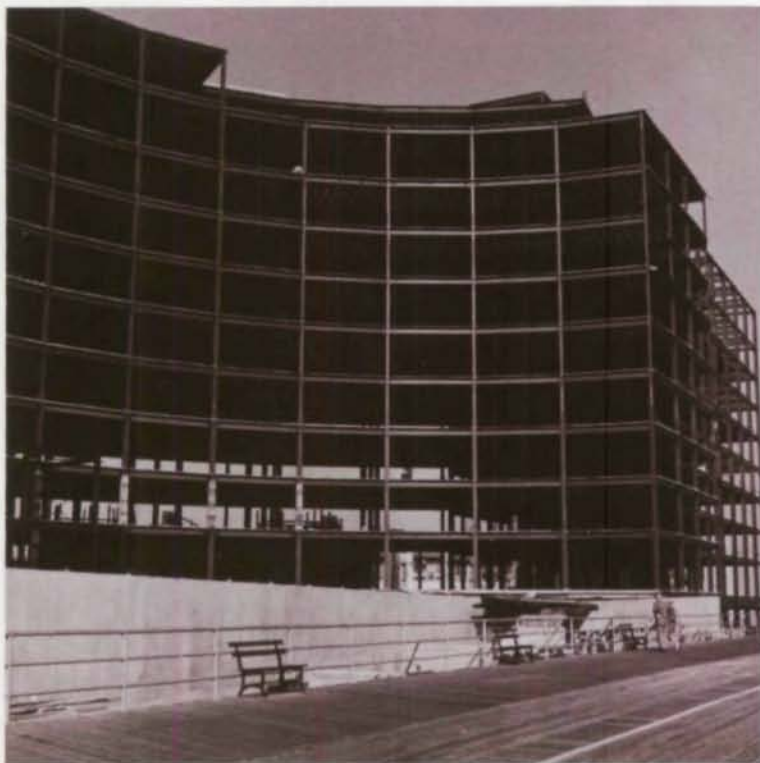
Steel framing saved 12.5% in construction of $4.5-million Ocean Manor Apartments on Atlantic City boardwalks.
