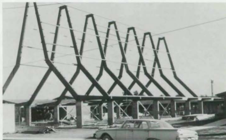
Economical in time and money, bents were fabricated in two pieces and field connected.
