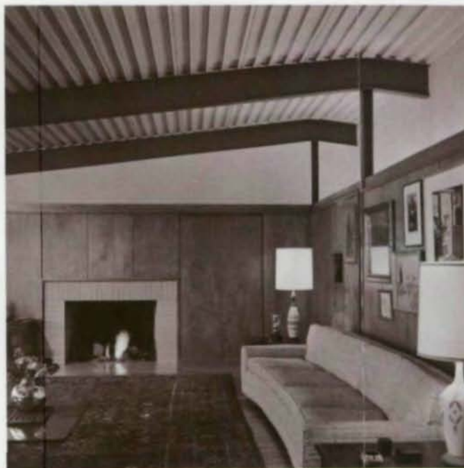
Crisp lines of exposed steel beams and decking emphasize and complement warm feeling of wood.
