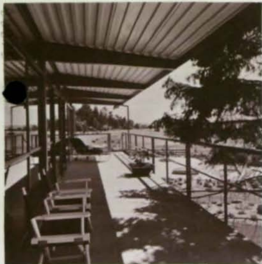
Steel frame eliminates need for load-bearing walls, permits broad view of nearby Puget Sound.
