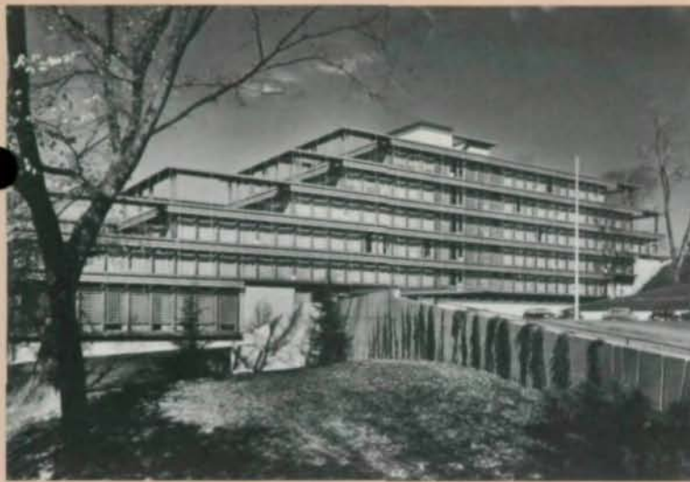
Chancery for the Federal Republic of Germany Washington, D. C. Architect: Egon Eiermann
