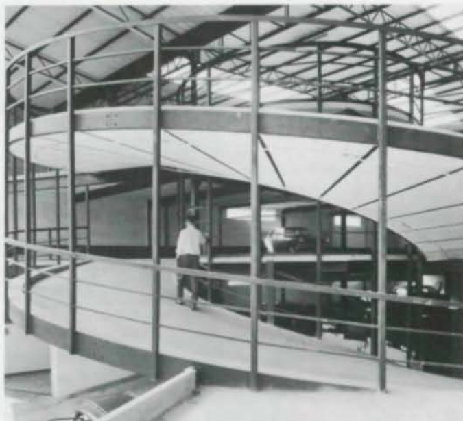
Photo courtesy of Acier Stahl Steel
