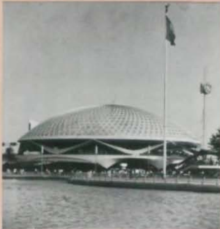
General Electric Progressland Pavilion New York World's Fair, New York Architect: Welton Becket and Associates
