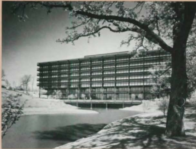
Deere & Company Administrative Center Moline, Illinois Architect: Eero Saarinen and Associates
