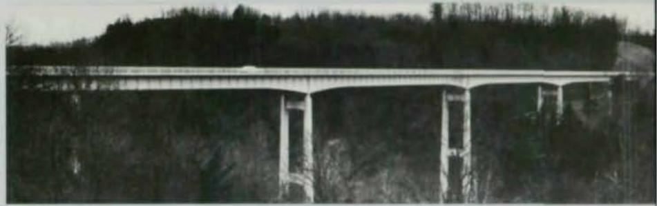
AWARD OF MERIT – MEDIUM SPAN, HIGH CLEARANCE Roanoke River Bridge, Blue Ridge Parkway, Roanoke County, Virginia Designer: U. S. Bureau of Public Roads Owner: National Park Service, U. S. Department of Interior General Contractor: McDowall and Wood, Inc. Fabricator: American Bridge Division – United States Steel Corp.
