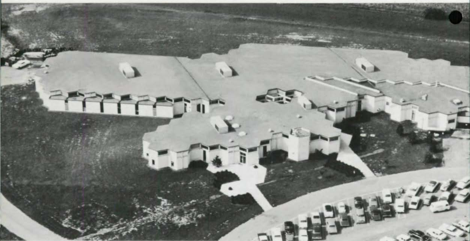
Flexibility was the key to the design of the Uniform Tubes plant. Result was an amoeba-like pattern based on a 192 sq ft hexagonal module.
