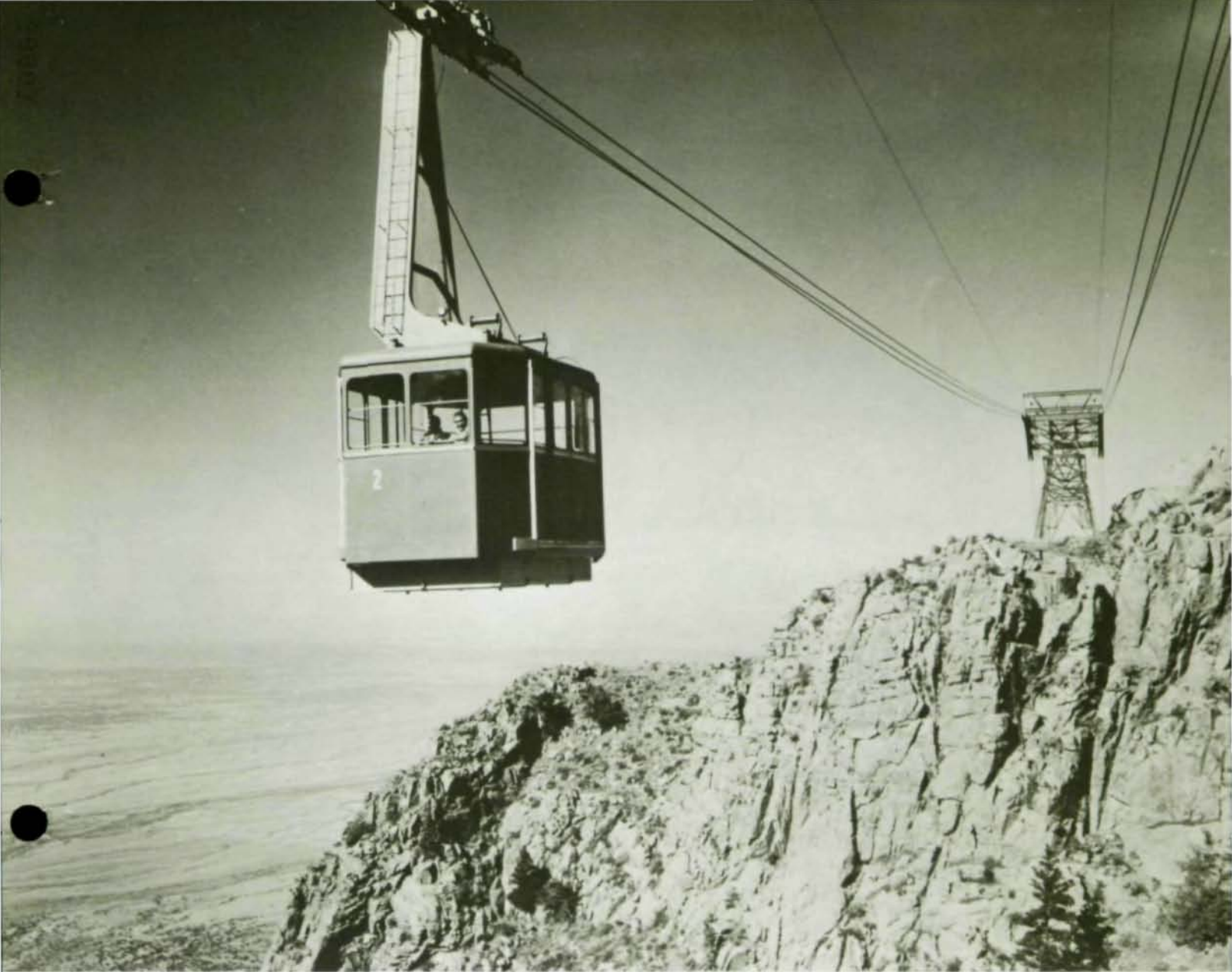
At one point the 60-passenger cabin of the tramway soars 1,400 ft off the ground. In the right background is Tower No. 2.
