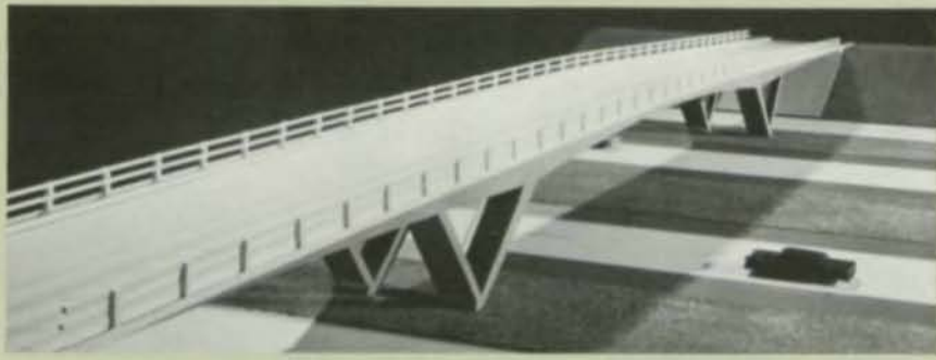
Combined engineering talent of two students from Denmark produced this design for a three-span steel highway bridge judged the Second Student Award winner. The students are Jorgen Gimsing and Peter Engberg, both 1966 graduates of the Technical University of Denmark. The bridge is a continuous box-girder structure. It features interior delta columns integral with the twin superstructure box girders and inclined away from the main traffic lanes. The two-box girders act compositely with a reinforced concrete deck, are six feet wide and have a variable depth.
