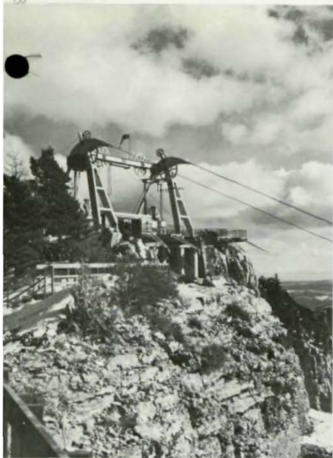
The breakovers at the summit support 224 tons of track cables.
