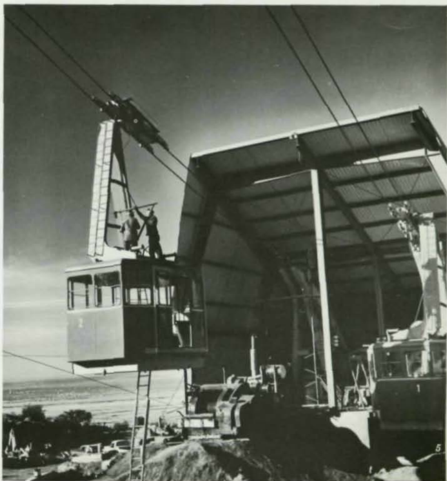
Workmen install the two 60-passenger cabins at the lower terminal.
