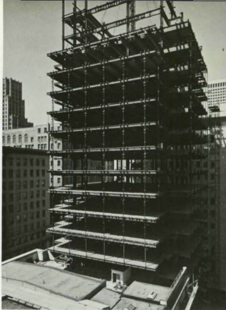
New framing cantilevers 29 feet into air space over the landmark 1908 building. Cantilevers on three sides provide floor space equivalent to 9 additional stories.
