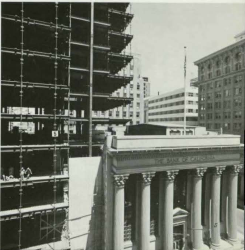
New framing cantilevers 29 feet into air space over the landmark 1908 building. Cantilevers on three sides provide floor space equivalent to 9 additional stories.
