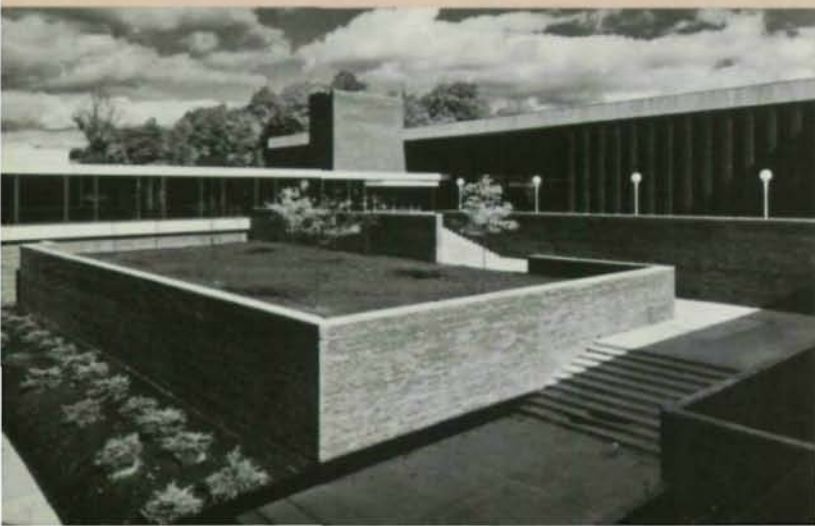
WHITESBORO SENIOR HIGH SCHOOL, Whitesboro, New York Architect: The Perkins & Will Partnership and Frank C. Delle Cese
