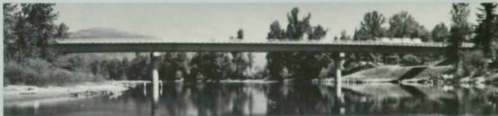
▶ AWARD OF MERIT – MEDIUM SPAN, LOW CLEARANCE Woodland Bridge Woodland, Washington Designer: Bjorn A. Stiansen, Harry R. Powell & Associates Owners: Cowlitz County and Clark County, Washington General Contractor: Ralph Lockyear Construction Co. Steel Fabricator: Fought & Company, Inc.
