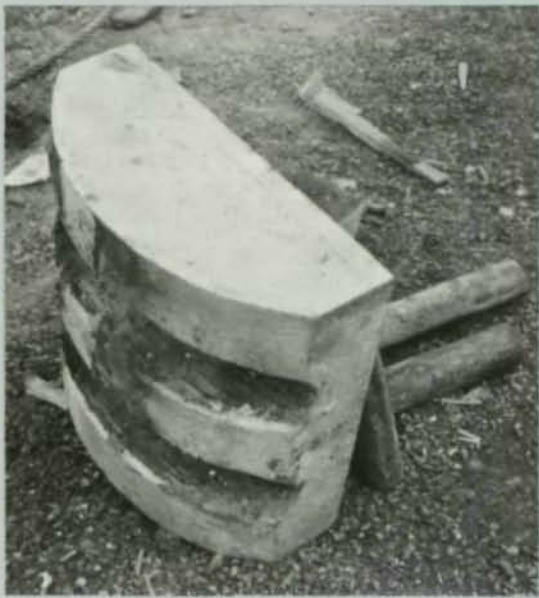
Cast iron cable saddle and roller assembly.
