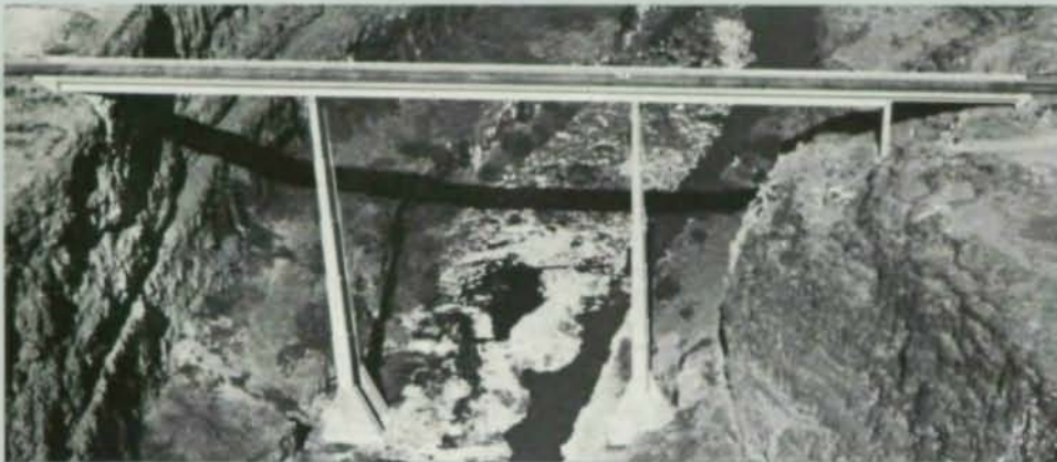
◀ AWARD OF MERIT – MEDIUM SPAN, HIGH CLEARANCE Hansen Bridge Over Snake River near Hansen, Jerome and Twin Falls Counties, Idaho Designer: Idaho Department of Highways (Bridge Section) Owner: Idaho Department of Highways General Contractor: Peter Kiewit Sons Company Steel Fabricator: Western Steel Company
