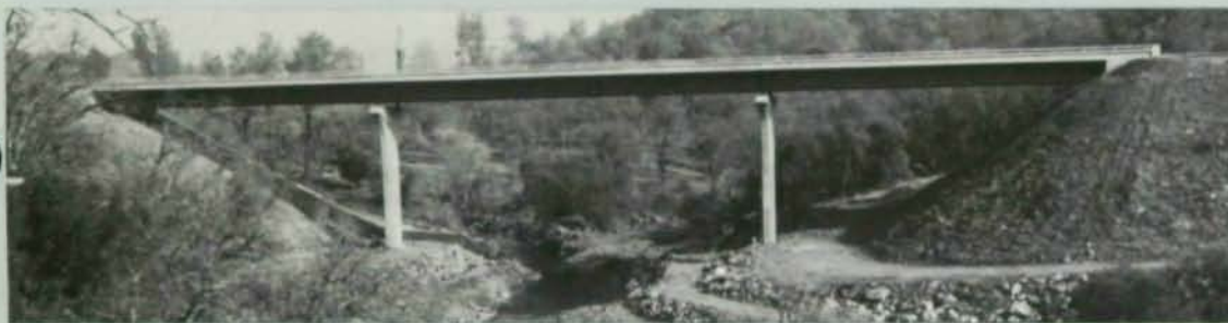
◀ AWARD OF MERIT – SHORT SPAN Dry Creek Bridge Ione, California Designer: State of California Bridge Department Owner: State of California General Contractor: O. K. Mittry & Sons and A. L. Croft (Joint Venture) Steel Fabricator: San Jose Steel Co., Inc.
