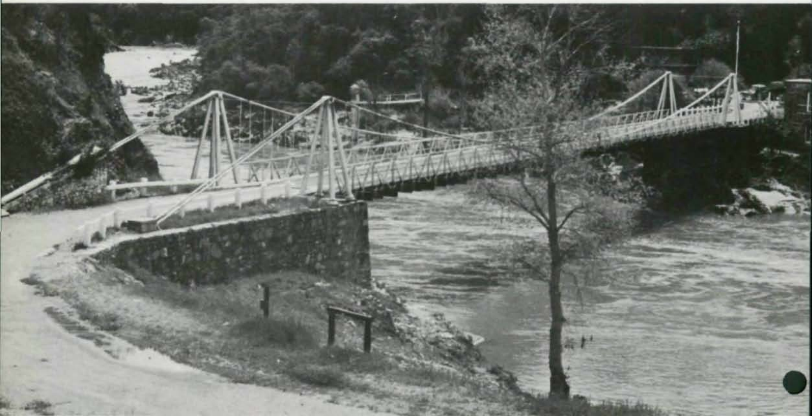
Bridge and toll house before dismantling.
