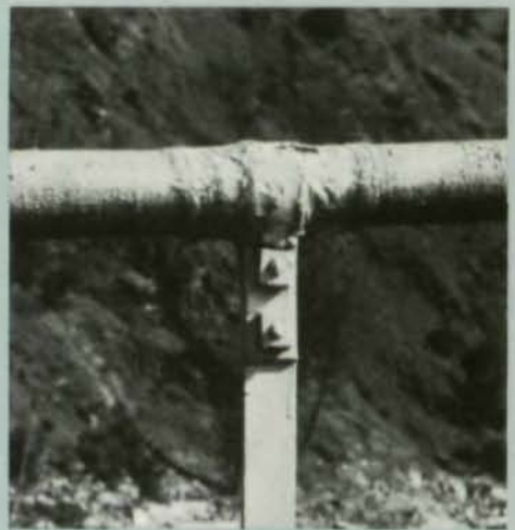
General appearance of cables throughout the bridge.
