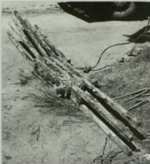
Anchor assembly of wrought iron bars and pins. Little or no corrosion was noted even though these bars were buried for 110 years.
