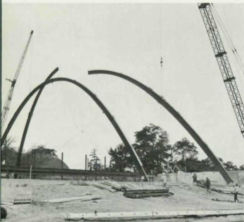
Steel arches were fabricated, shipped and erected in one-half sections. Spacer braces were removed after installation of roof planking.
