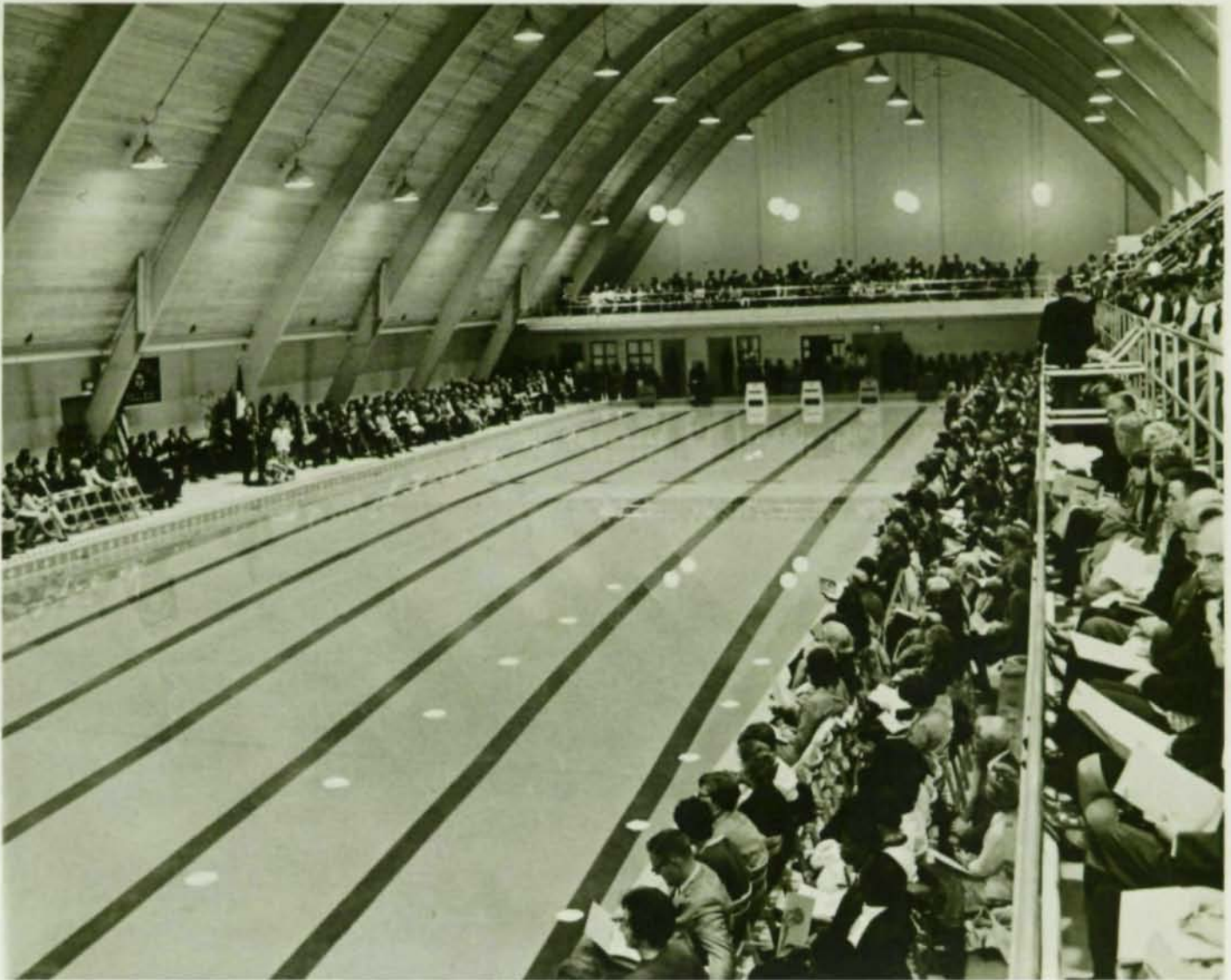
Exposed steel arches provide a graceful frame for indoor swimming pool. Repainting will not be required for 8 to 10 years.
