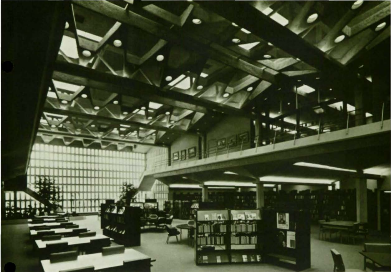
Steel roof trusses and bracing, fireproofed with lightweight cement plaster, create an unusual sculpture in space over the main reading area.
