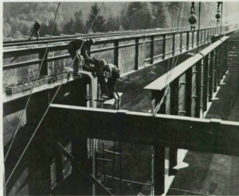
Aesthetic studies led to the choice of a welded plate girder bridge with uniformly tapered piers. Corrosion-resistant steel shells serve as permanent forms for concrete piers.
