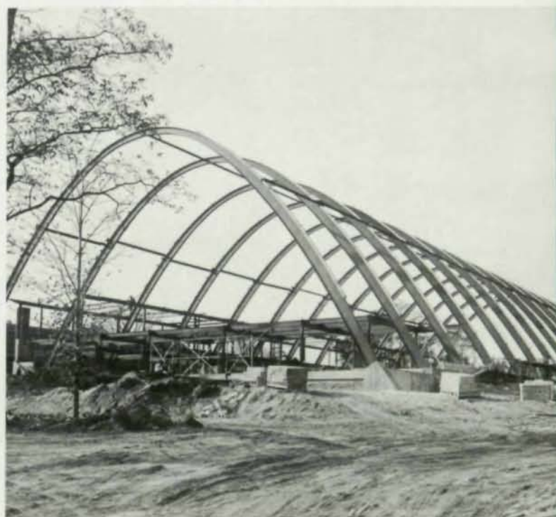
Steel arches were fabricated, shipped and erected in one-half sections. Spacer braces were removed after installation of roof planking.
