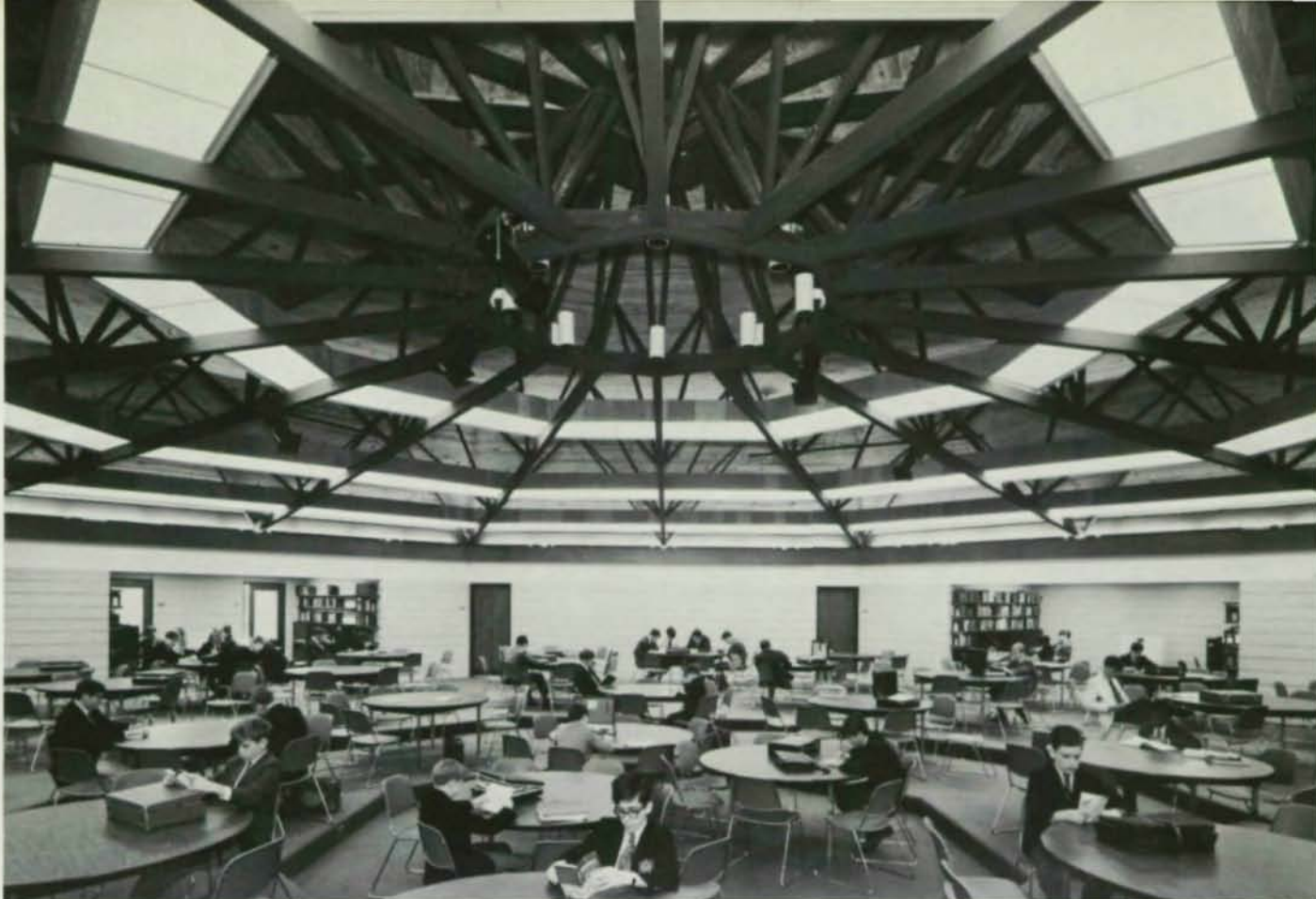
Tubular steel "V" trusses span the 72-ft octagonal central research-study area. The three-dimensional framing has an upper compression ring and a lower tension ring at the center.
