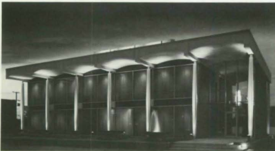
Each tapered column section is made up of four identical tee sections welded stem to stem. The tees were cut from 12WF27 sections, as illustrated.
