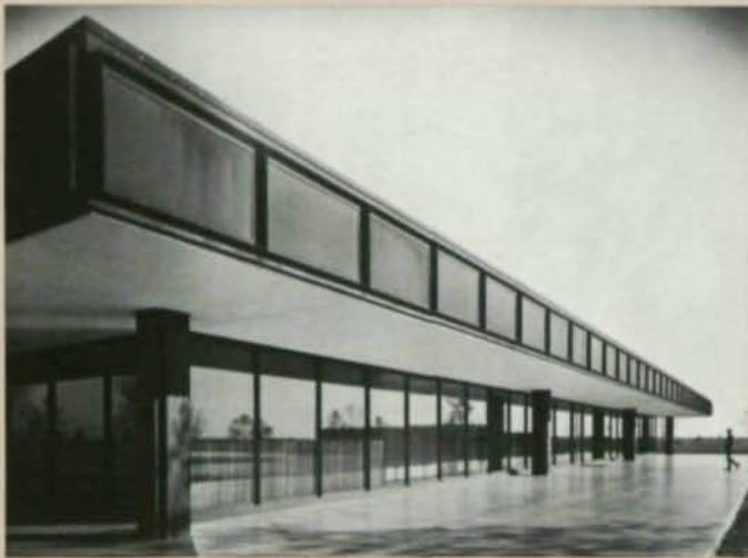
SUPERIOR OIL COMPANY GEOPHYSICAL LABORATORY , Houston, Texas Architect: Todd-Tackett-Lacy, Architects & Planning Consultants
