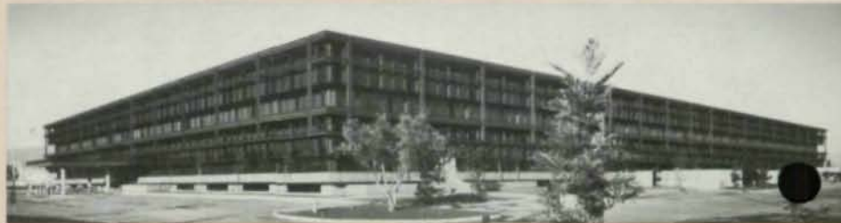
FAIRCHILD SEMICONDUCTOR HEADQUARTERS BUILDING , Mountain View, California Architect: Simpson, Stratta & Associates
