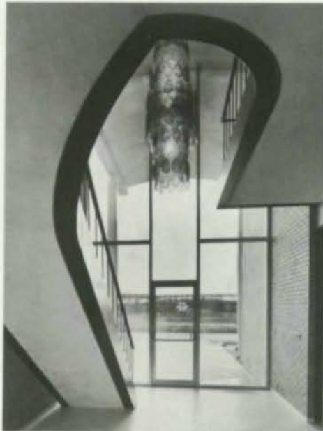
The semicircular stair at the entry is designed with steel box stringers, requires no intermediate support between floors.
