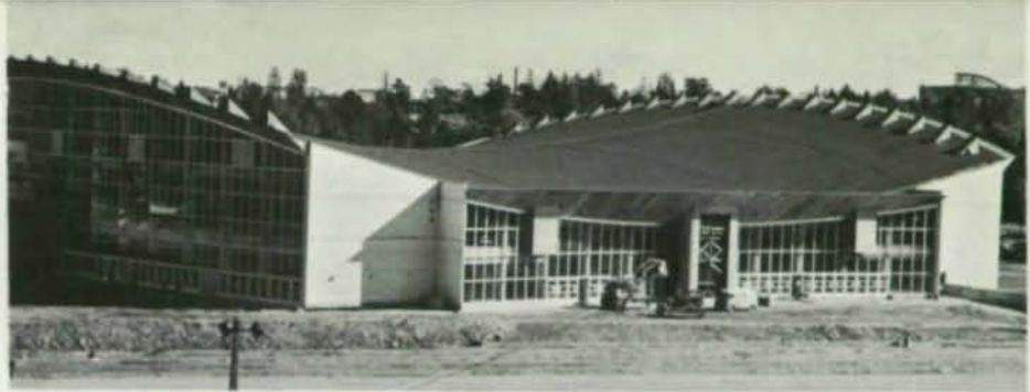
The cable roof of the Helsinki Ice Stadium spans 240 ft. Note that the roof line follows the curvature of the cable trusses.
