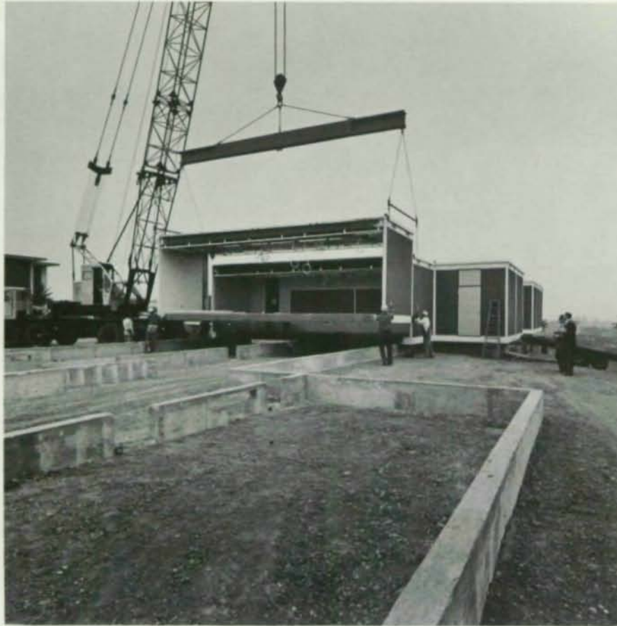
After modules were manufactured, they were moved to site and lifted by crane onto previously constructed footings.
