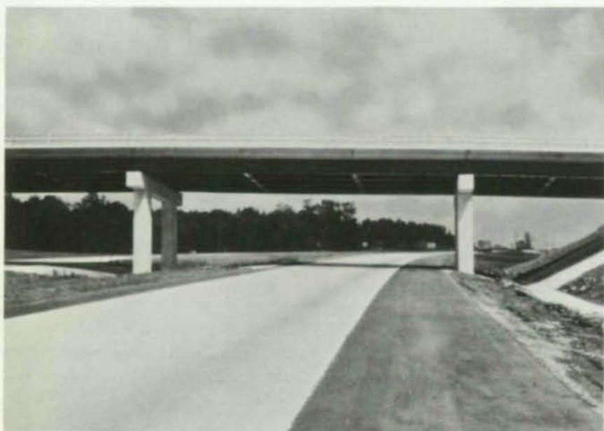
Prize winning two-span steel beam overpass in San Bernardino County, California has no side piers. Three-span structure requires bents very close to traveled way, causing unnecessary hazard to motorists.
