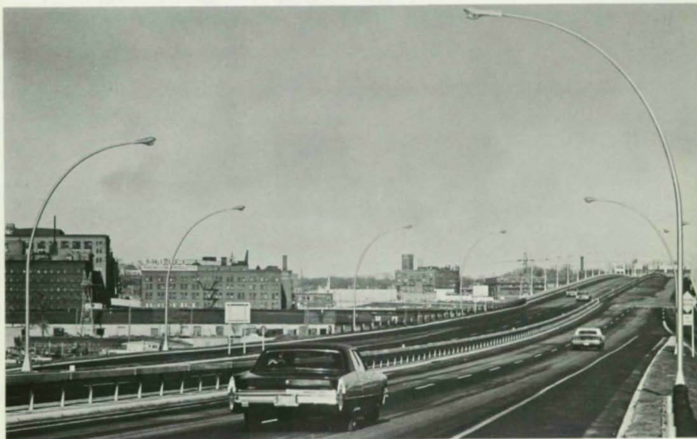
Two 29-ft roadways, each with two lanes of traffic, are separated by a 4-ft wide raised median at the center.
