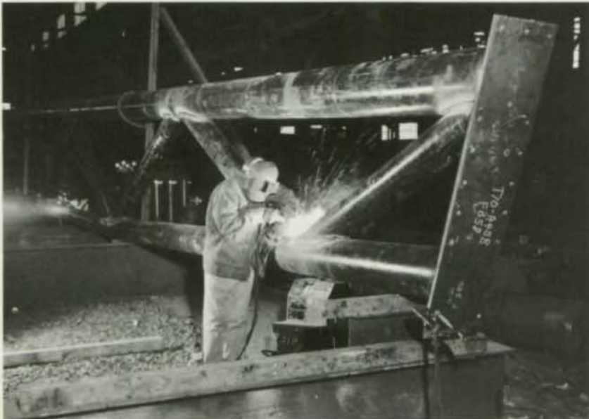
Photos from Lincoln Arc Welding Foundation
