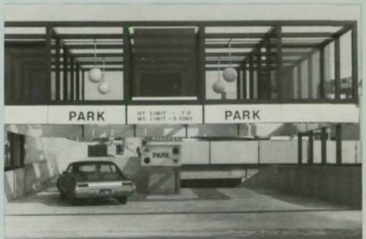
AIR RIGHTS PARKING DECKS — ENTRANCE CANOPIES , Atlanta, Georgia Architect: Toombs, Amisano and Wells, Architects
