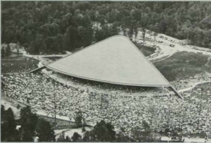
BLOSSOM MUSIC CENTER , Northampton Township, Ohio Architect: Schafer, Flynn, van Dijk, and Dalton, Grimm, Johnson
