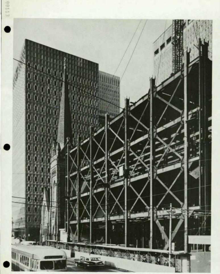
Use of X-bracing members (ASTM A514 - 100,000 psi yield strength) reduced drift to a minimum.
