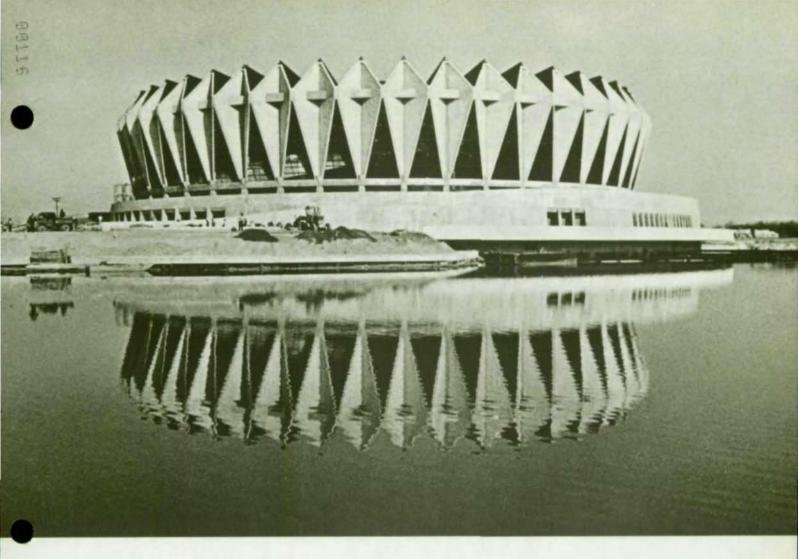
The design of the recently dedicated \$6.8-million Hampton Roads Coliseum, in Hampton, Va., was inspired by the symbol of the Tidewater area — white sails. Exterior sail-shaped wall panels support a 400-ft dia. cable-suspended clear span roof.
