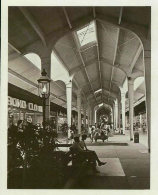
The design of the bents achieves a high spacious volume through the center of the mall and creates more intimate walkways of comfortable scale along the storefront shopping areas. Skylights are used intermittently to form pools of daylight and various light intensities for interest and accents.
