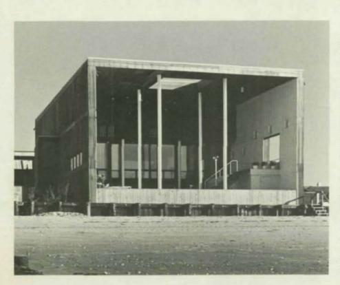
High waves can crash into the Spatrium and flow out under the house unobstructed. The wind can pass freely into the Spatrium and escape through openings in the shear walls and roof.
