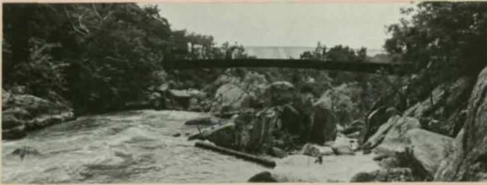
AWARD OF MERIT 1970 — SPECIAL TYPE Olmstead Island Footbridges Great Falls, Maryland Designer: U. S. Department of the Interior Owner: U. S. Department of the Interior General Contractor: Slavin & Shafer, Inc. Steel Fabricator: Leckenby Company
