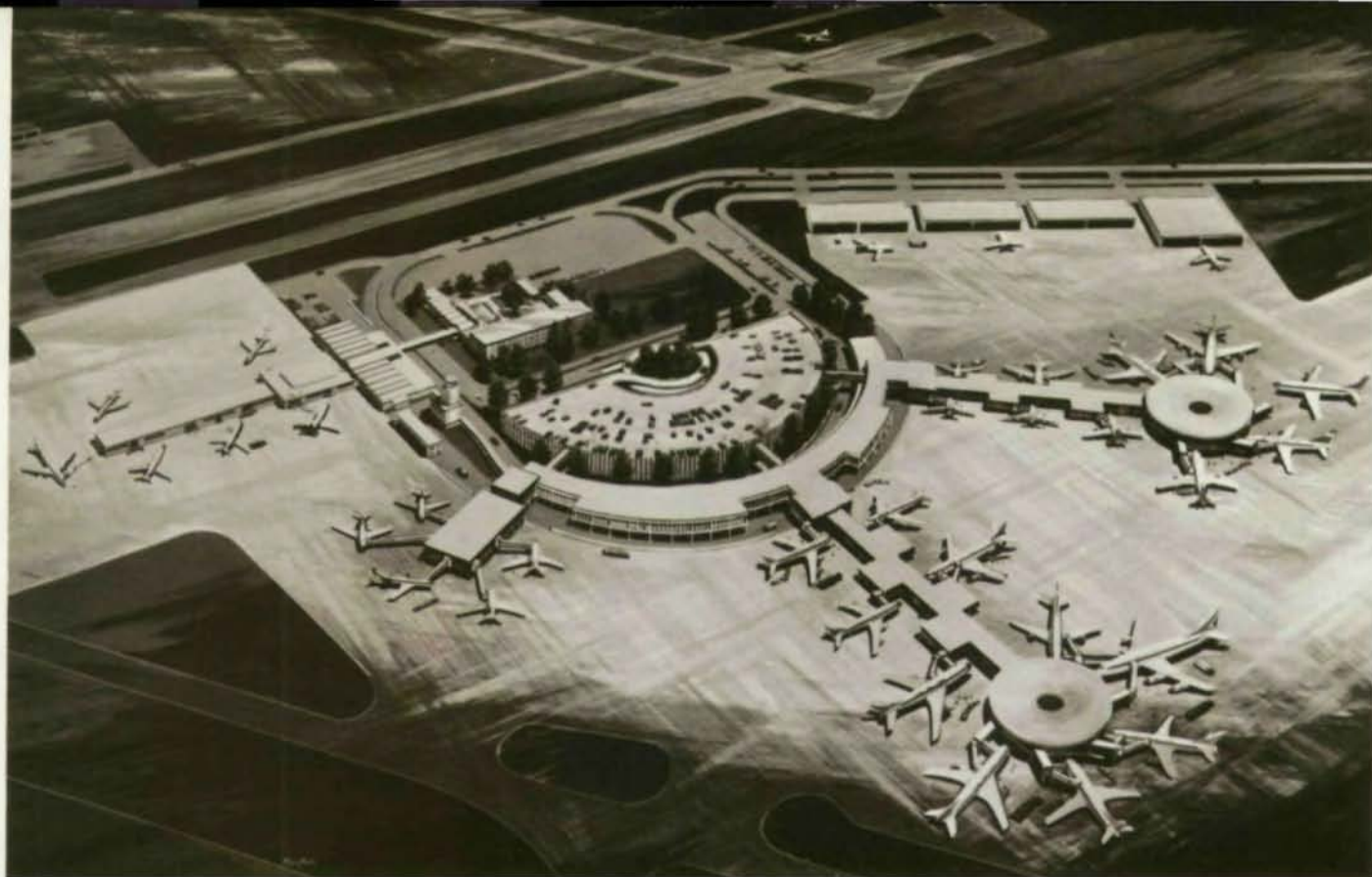
Birmingham's Municipal Airport will be one of the most modern airports in the nation.
