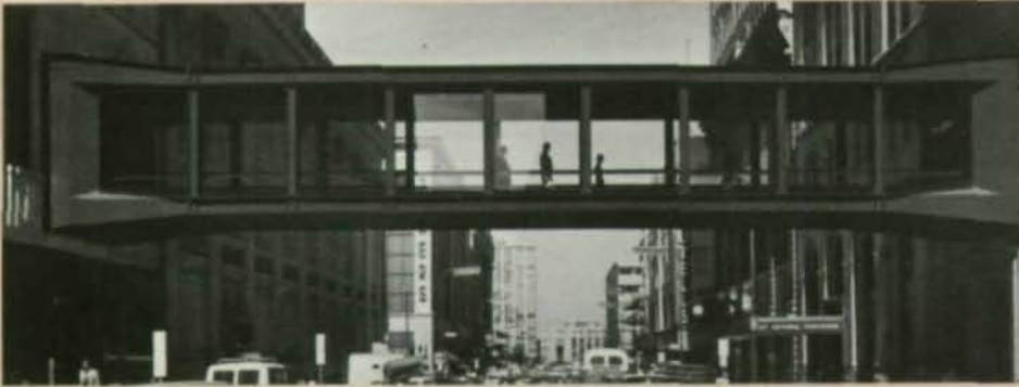
AWARD OF MERIT 1970 — SPECIAL TYPE Pedestrian Skyways Minneapolis, Minnesota Designers: The Cerny Associates, Inc. Meisch and Robertson Owners: Dain, Kalman & Quail, Inc. Farmers & Mechanics Savings Bank of Minneapolis Minnesota Federal Savings & Loan Association First National Bank of Minneapolis General Contractor: Naugle-Leck, Inc. Steel Fabricator: Crown Iron Works Company
