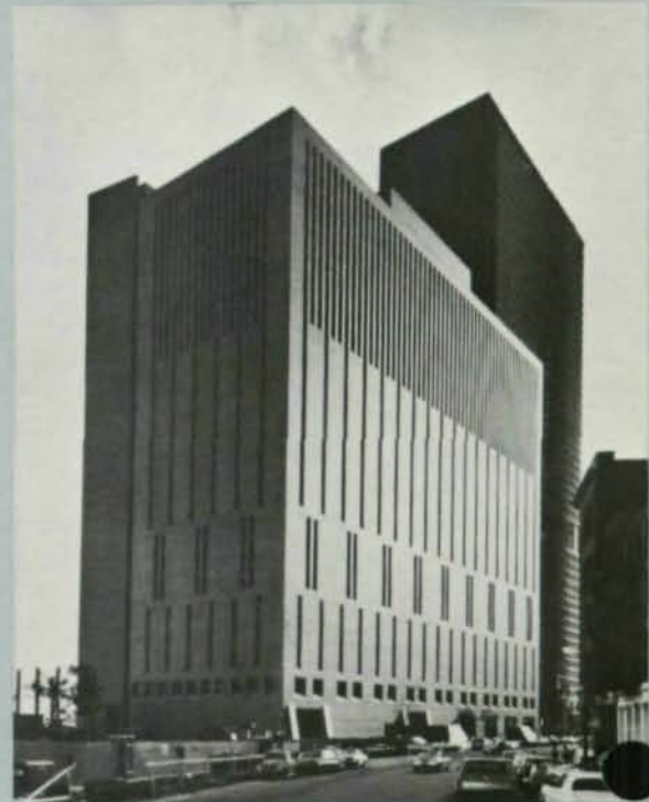
▼ MANUFACTURERS HANOVER TRUST CO. OPERATIONS BUILDING , New York, New York Architect: Carson, Lundin & Shaw
