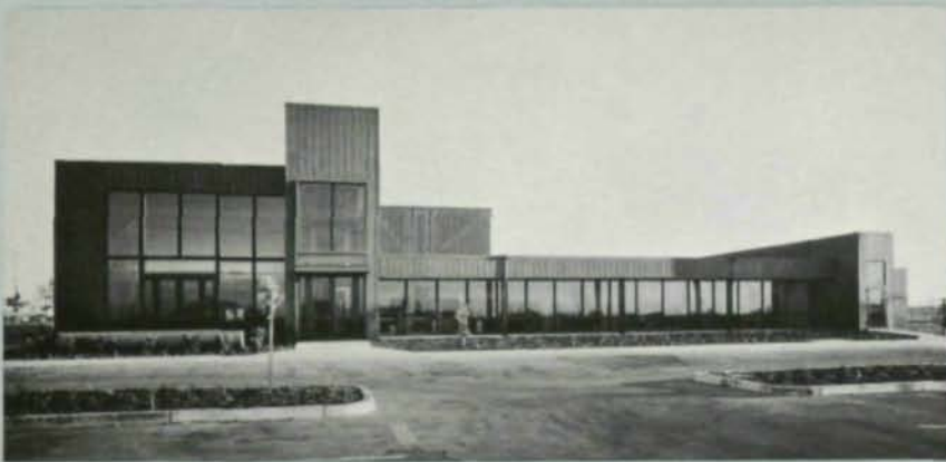
▲ GRT CORPORATE HEADQUARTERS BUILDING , Sunnyvale, California Architect: Brown/McCurdy/Nerrie
