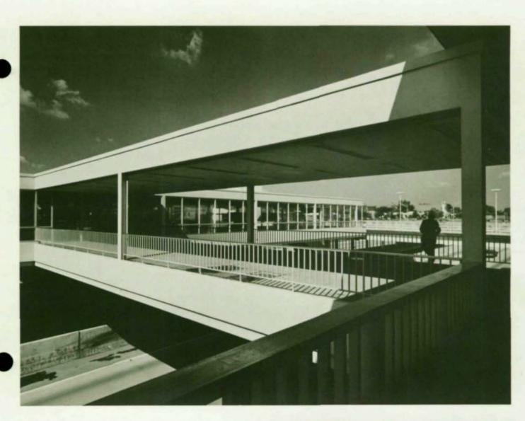
posed by structures of these types. Welded steel connections were used to give a finished appearance, and to obtain smooth surfaces. Finally, the architects were able to make the steel construction the basis of the architectural expression of the stations, since the building code permitted non-fireproofed steel in most cases.
