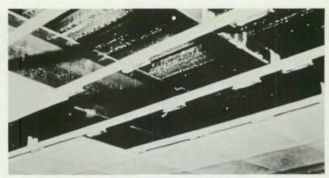
Fire-rated acoustic tile ceiling showing exposed steel decking and beam
