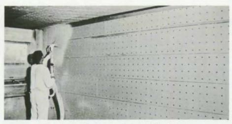
Plasterer spraying basecoat over perforated lath on wall
