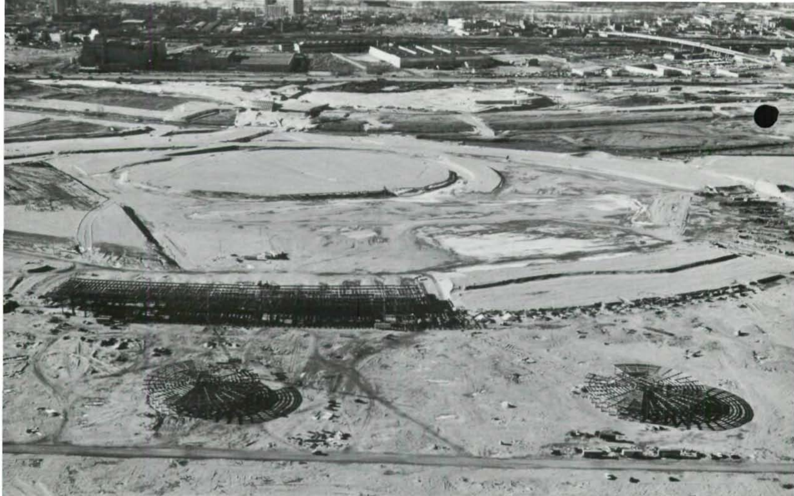
Aerial view of terminal building and two satellites
