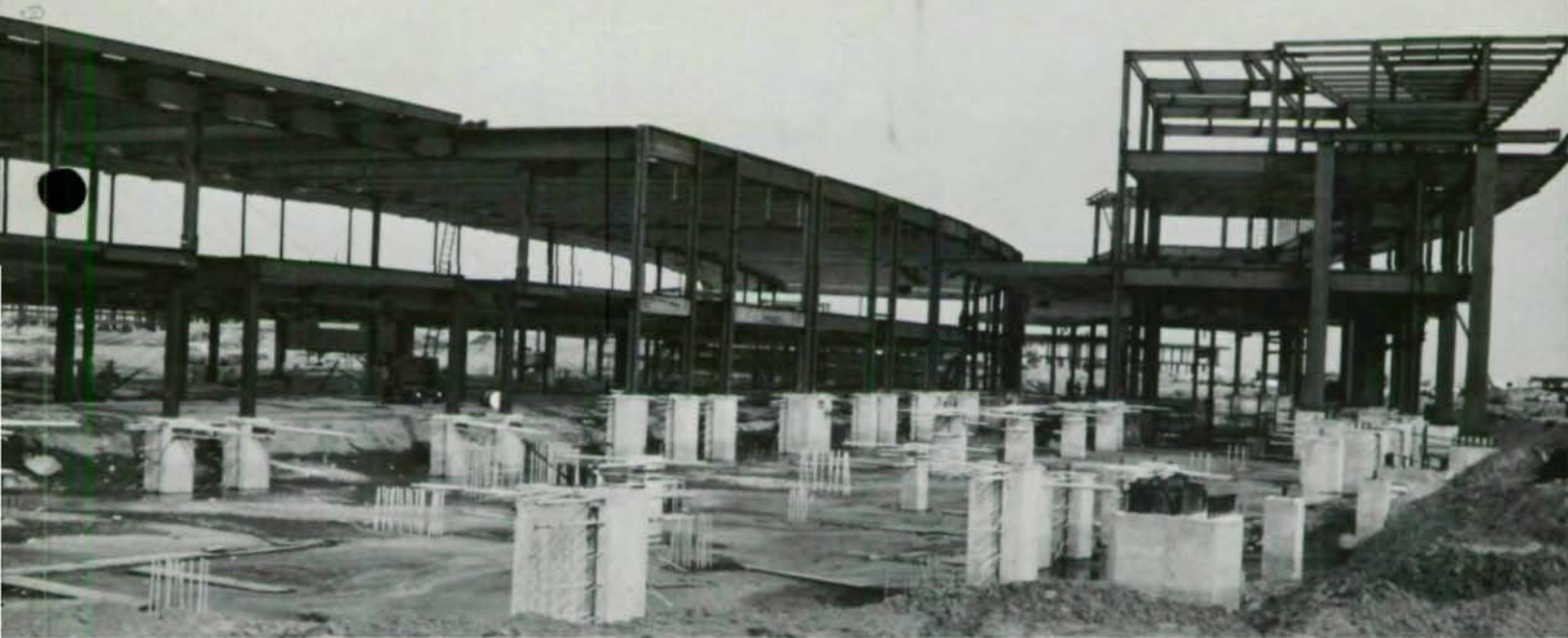
Steel framing for Main Building
