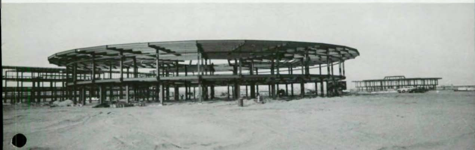
Steel framing of one of nine satellite buildings
