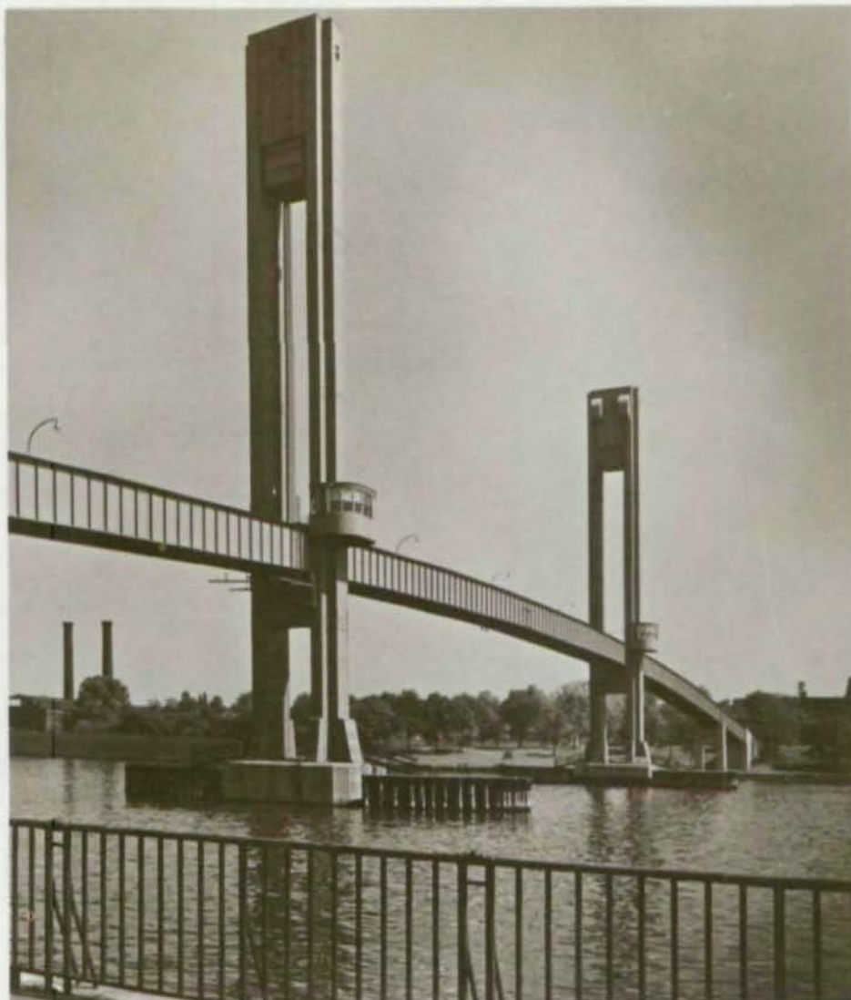
The Harlem River Pedestrian Bridge
