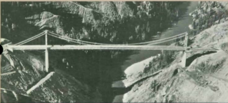
AWARD OF MERIT 1972 — LONG SPAN Dent Bridge Clearwater County, Idaho Designer: Howard, Needles, Tammen & Bergendoff Owner: U. S. Army Corps of Engineers General Contractor: Hensel Phelps Construction Co. Steel Fabricator: Fought & Company, A Division of Allied Equities Corporation
