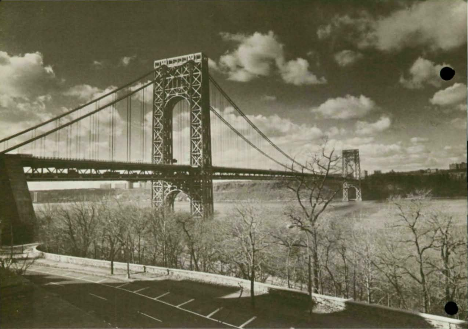
The George Washington Bridge
