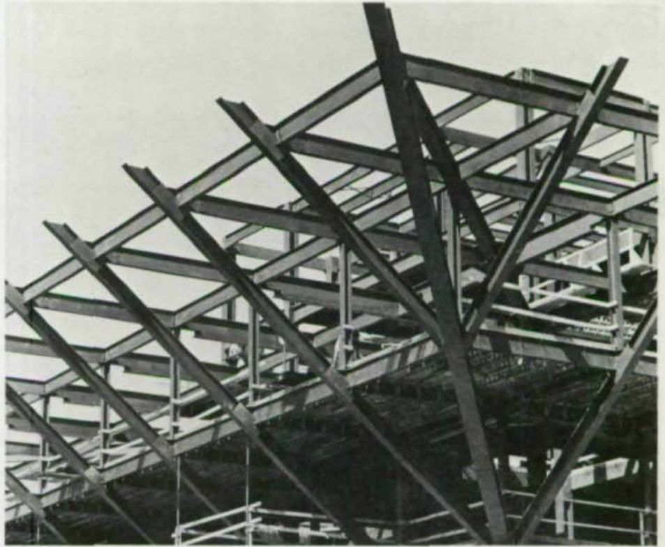
The corner diagonals support up to a 500 ton load.
