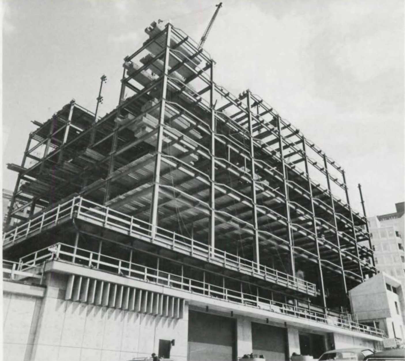
The John McCormack State Office Building has realized savings in time and money by selecting structural steel.
