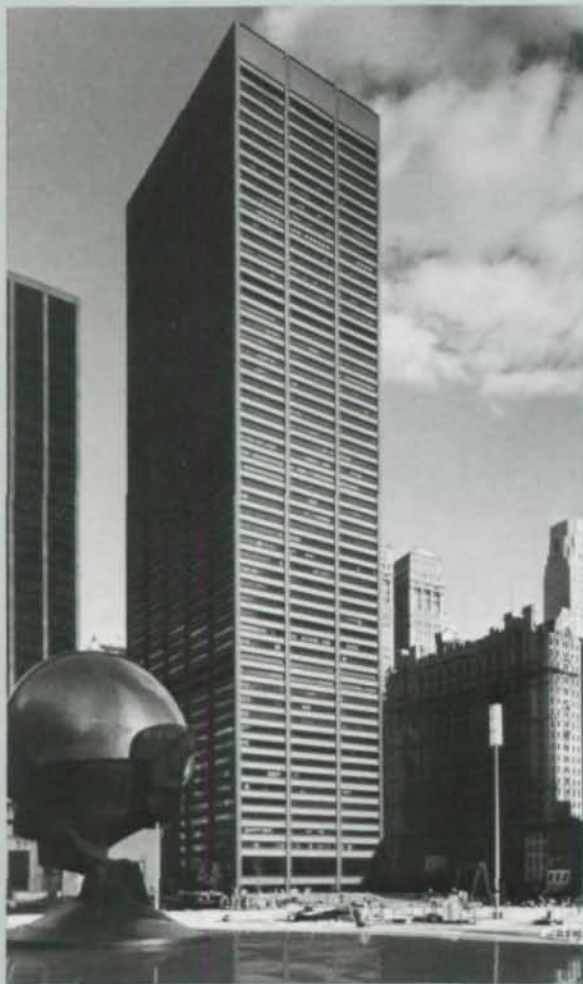
▲ ONE LIBERTY PLAZA New York, New York Architect: Skidmore, Owings & Merrill
