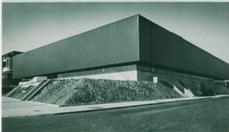
The Broome County Veterans Memorial Arena provides 7,000 seats for spectators and floor area for sports, shows, conventions, and other exhibitions. A separate adjacent gallery structure contains lobbies and meeting rooms.
