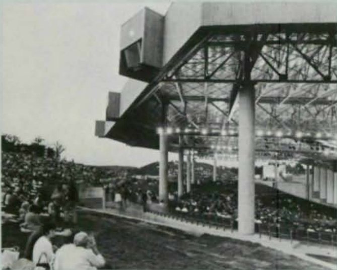
PINE KNOB MUSIC THEATRE Independence Township, Michigan Architect: Rossen/Neumann Associates
