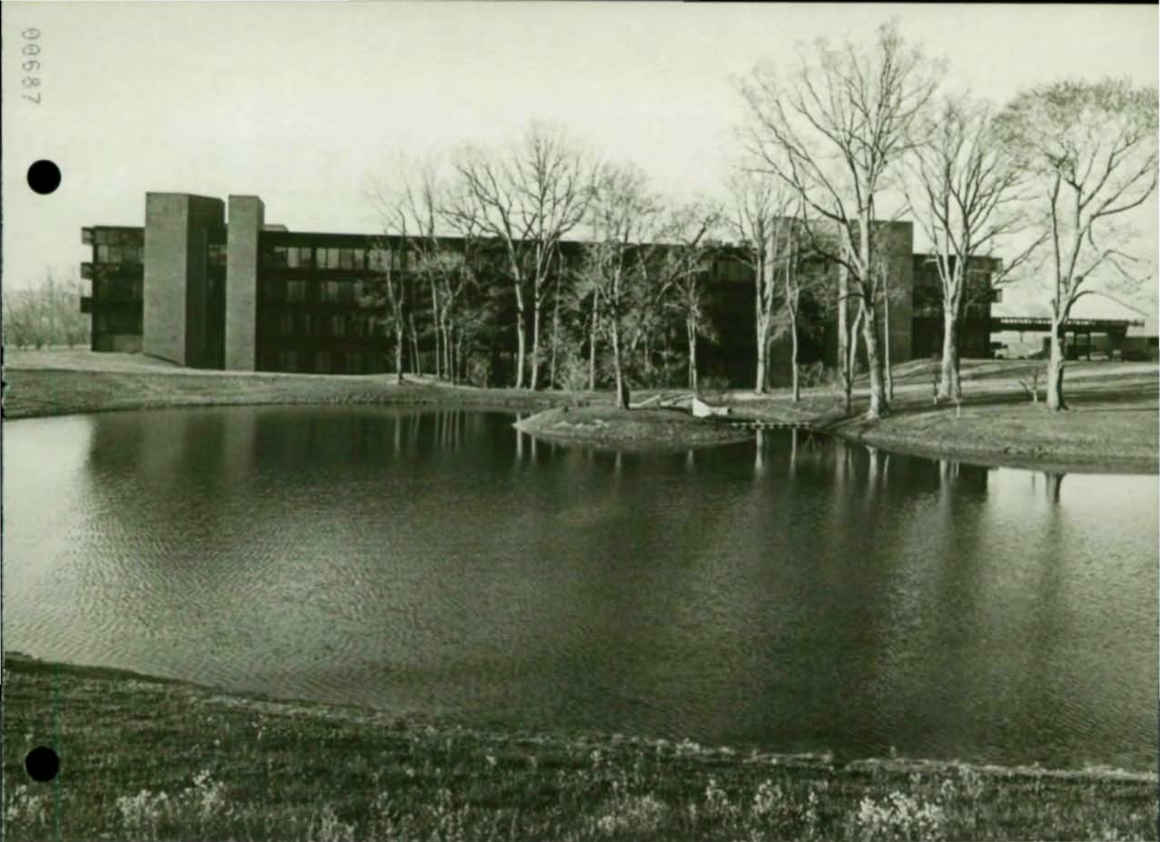
Weathering steel exterior columns and spandrels blend with the building's wooded setting.
