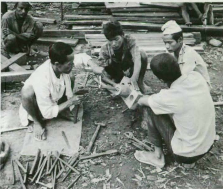
A technician on loan from the Nepal Ropeway "sockets" our bridge strand.
