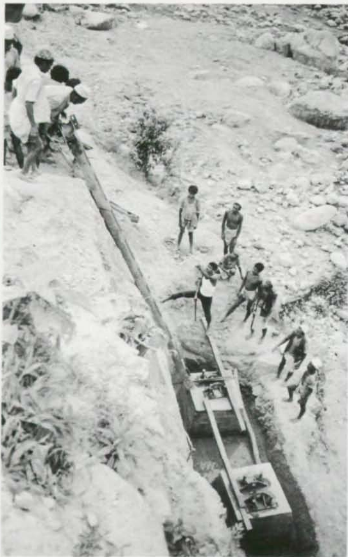
Work proceeds on west tower.
