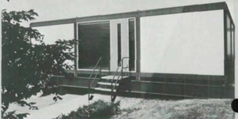
▶ CONTROL CENTER FOR POWER PLANTS Lawton, Oklahoma Pittsburgh, Pennsylvania Architect: Robert L. Ziegelman
