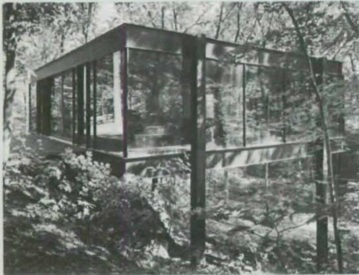
▲ STUDIO Highland Park, Illinois Architect: David Haid
