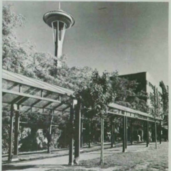
▼ SEATTLE CENTER COVERED WALKWAYS Seattle, Washington Architect: The Richardson Associates
