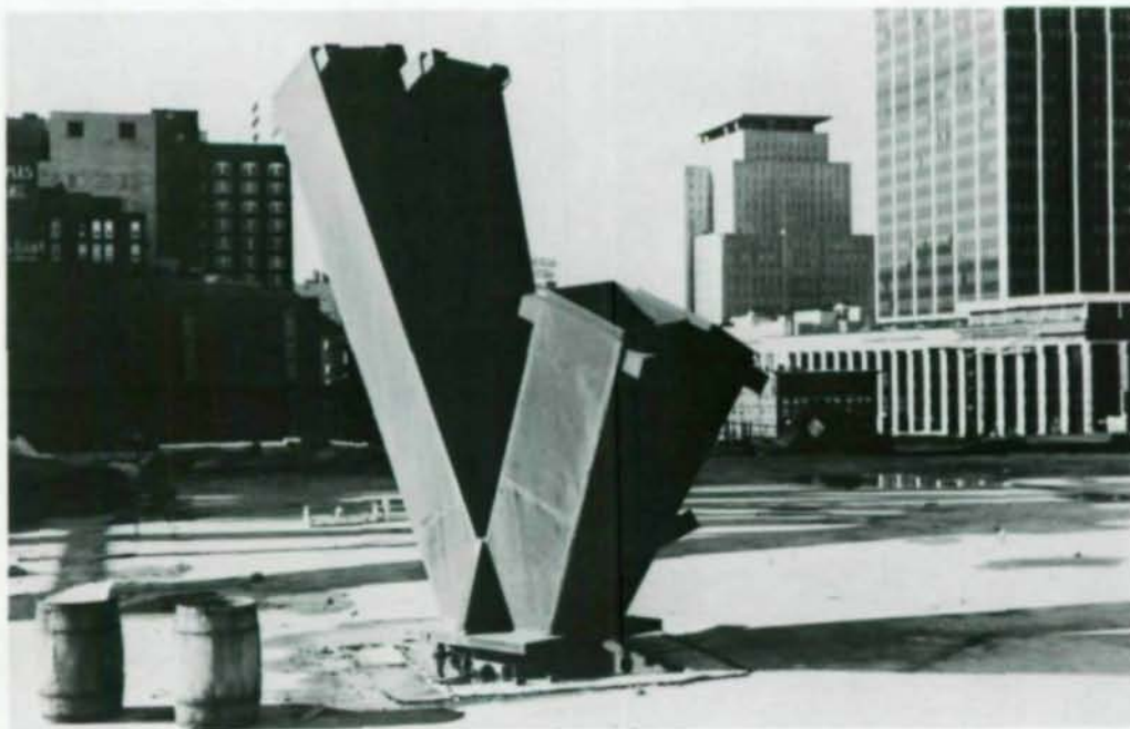
Typical four column "cluster" base erected with bearing in place.
