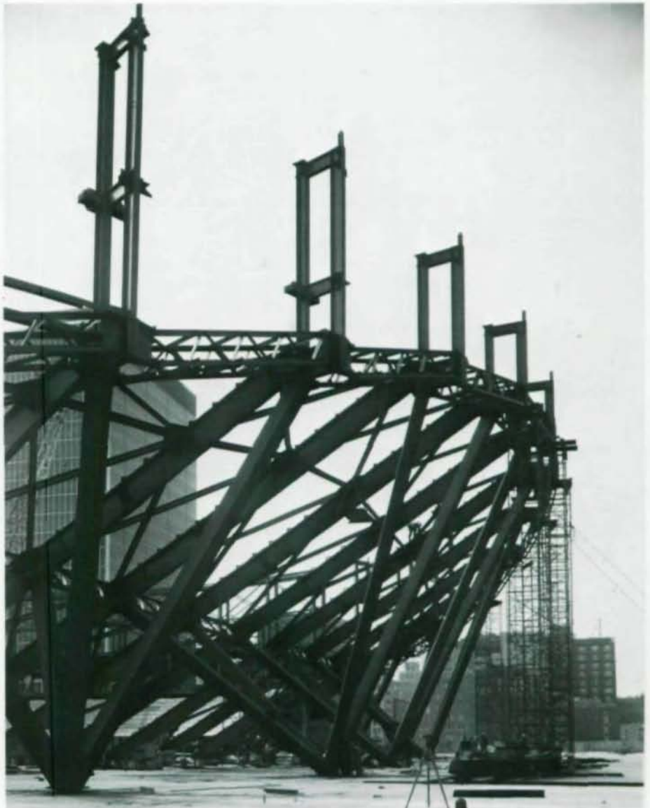
Space frame of north garage.
