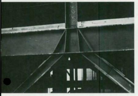
Again, the problem of severely restricted story heights becomes an immediate problem since there was no appreciable depth for a girder. It was also thought that the girders could be eliminated and the frame could span the two bays by vierendeel action. Or, as an analogy, it could be said that two larger holes were put in the wall of the tube. Subsequent computer analyses showed that selected columns could, with little increase in total weight, be eliminated.
