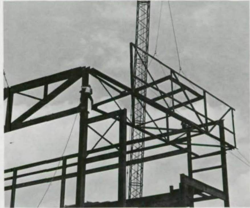
Erection of shop-assembled bracing trusses
