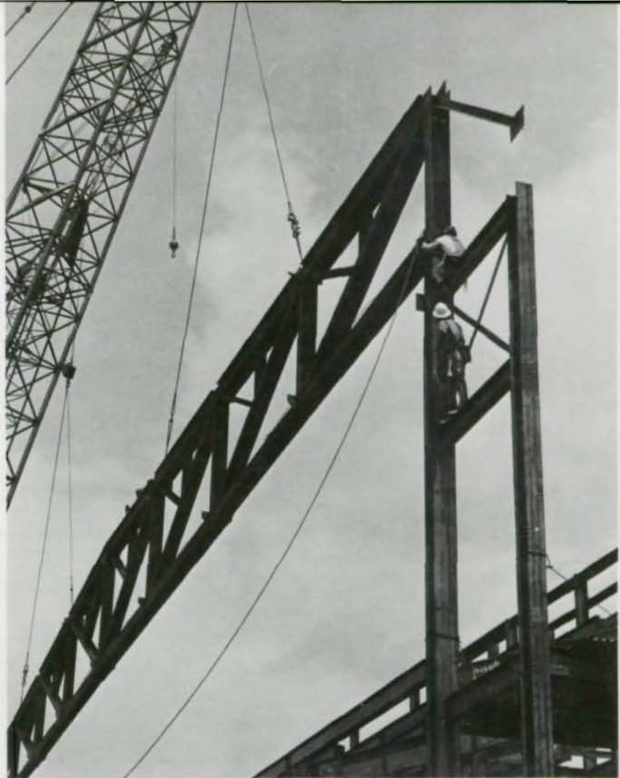
Seating end of first truss on rocker bearing
