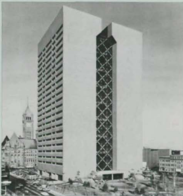
HENNEPIN COUNTY GOVERNMENT CENTER Minneapolis, Minnesota Architect: John Carl Warnecke & Associates ▼
