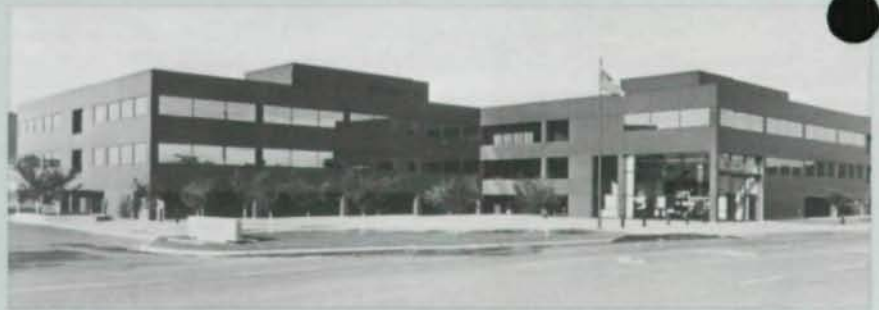
▶ FREIGHTLINER CORPORATE HEADQUARTERS Portland, Oregon Architect: Boutwell, Gordon, Beard and Grimes
