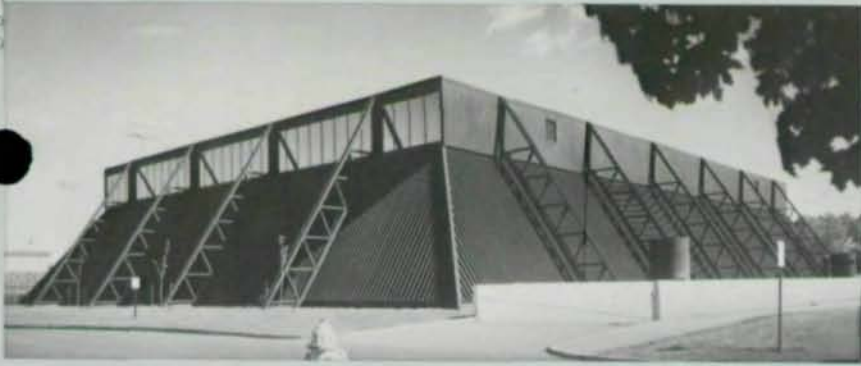
▲ PHYSICAL EDUCATION FACILITY UNIVERSITY OF MINNESOTA Duluth, Minnesota Architect: The Leonard Parker Associates
