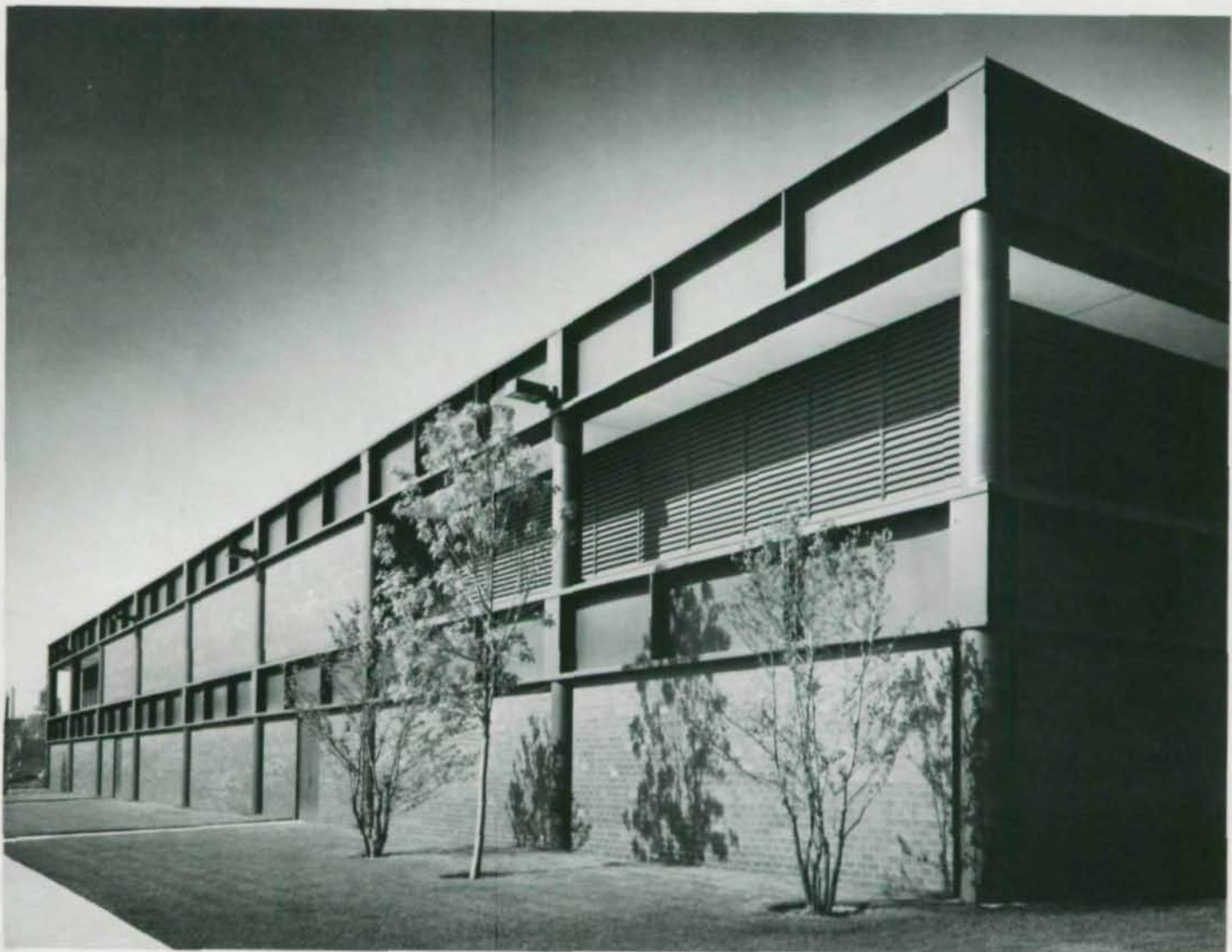
The exterior spandrels are steel plate girders, completely weather sealed to the column covers.
