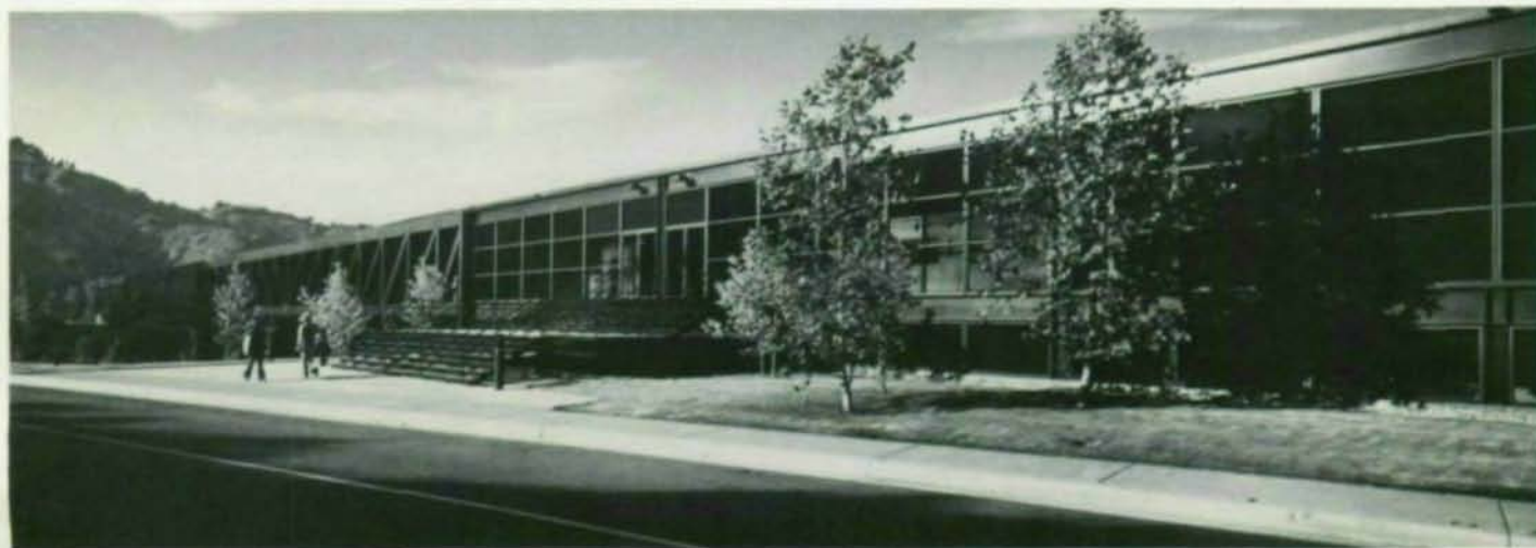
Two 2-story wings, both with one story below grade, contain classrooms and studies.
