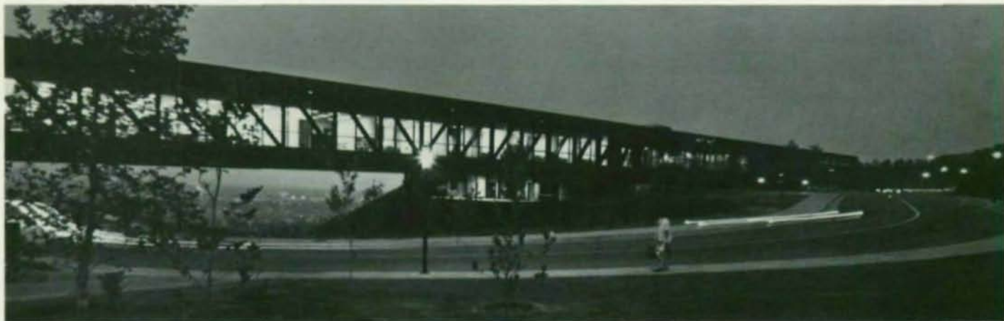
The entire bridge is supported by four 16-ft deep trusses.
