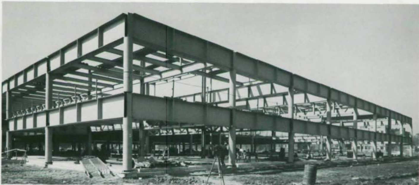
The structural steel system allowed for faster erection time.
