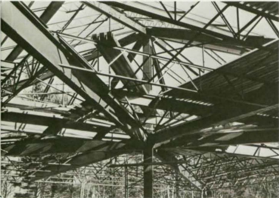
Steel truss system radiates from a central "maypole" column.
