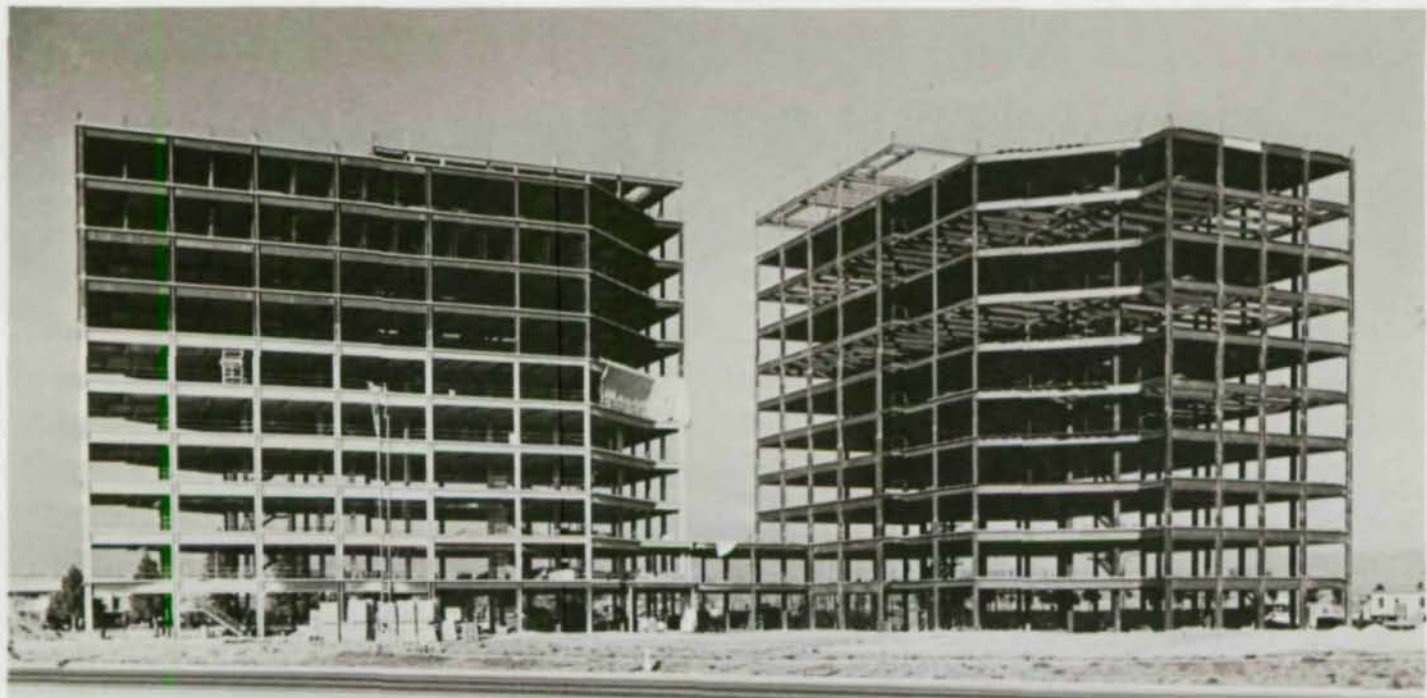
Height limitations led to a twin-tower design for KCN 10/10.
