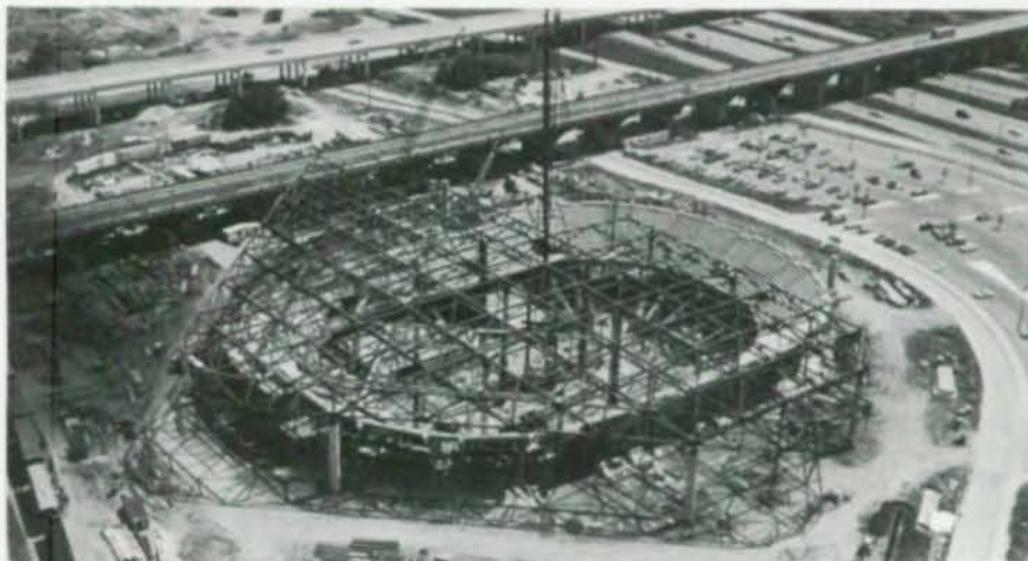
Aerial shows perspective of steel roof trusses to 17,200-seat arena.
