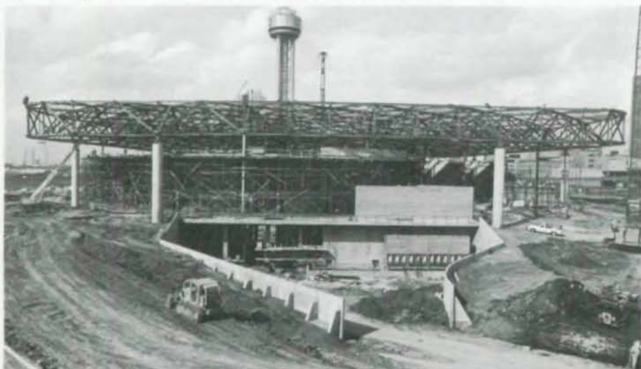
Topped out, gigantic steel space frame is ready for roof deck.
