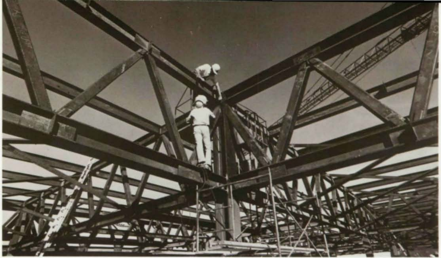
Erectors check trusses on second-floor interstitial level planned to facilitate mechanicals.
