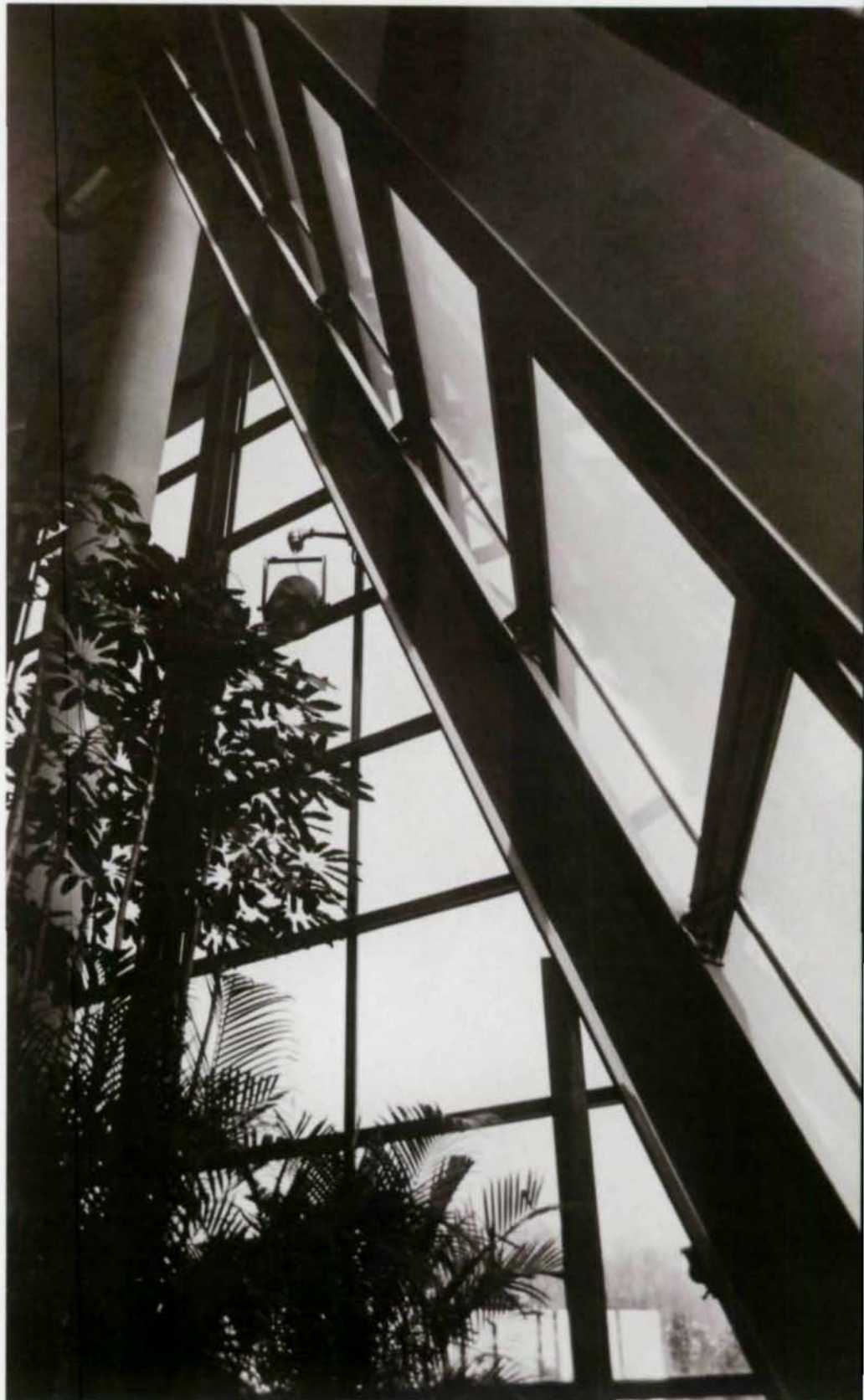
Steel members, and even high-strength bolts, remain exposed for strong visual effect.
