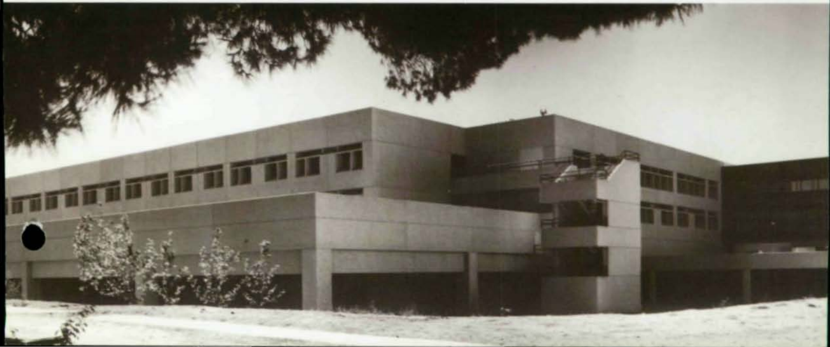
Newest St. Mary's addition on Arizona's oldest hospital turned growth to site center (see plan, l.). Tucson hospital was first one designed to meet 1976 seismic codes.
