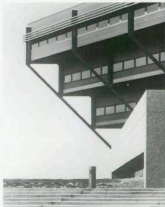
Striking "steps" contribute to both building's architecture and energy efficiency, major consideration in structure designed to recapture computer heat.
