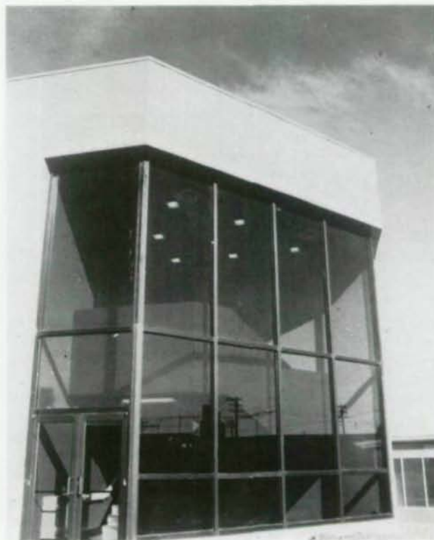
Glassed-in stairwell adds openness. Lightweight steel skin lends strong visual image to hospital.
