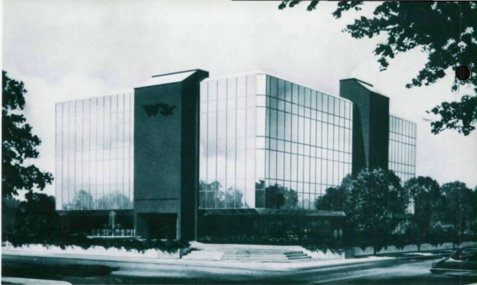
New Woonsocket Institution for Savings' corporate headquarters designed to attract commercial neighbors.
