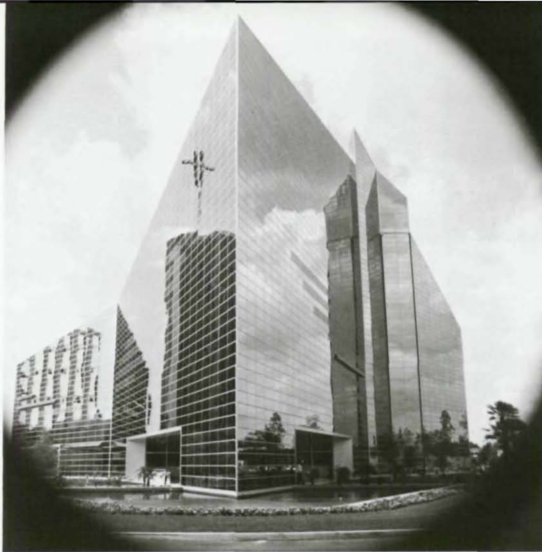
New home of Garden Grove Community Church, Crystal Cathedral reflects surroundings in sea of mirrors. Steel framework (below) details masterpiece of steel structure before it was sheathed in glass.
