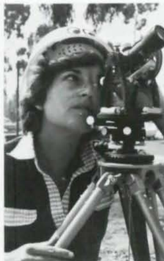
One of Pittsburgh-Des Moines Steel Company's field engineers, Nancy Bendel (l.) confers with ironworkers V.L. Cosgro and V.G. Kripal on critical details of erection. Eye on detail, Nancy checks close tolerances required to get sub-assemblies to fit precisely. Often four transits were working simultaneously.
