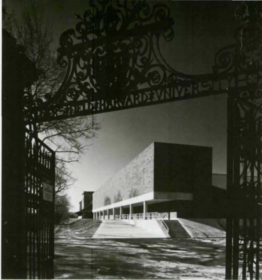
Traditional gate to Harvard University Athletics Complex swings open to new, contemporary Natatorium building. Photos by Nick Wheeler.
