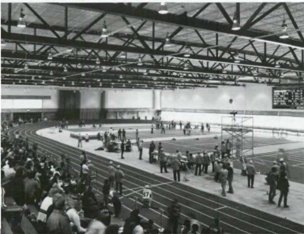
Largest clear-span trusses (12 ft x 192 ft) in New England bridge running tracks, infield tennis and weight-throwing areas and bleachers for 1,500 in new Track & Tennis Hall.
