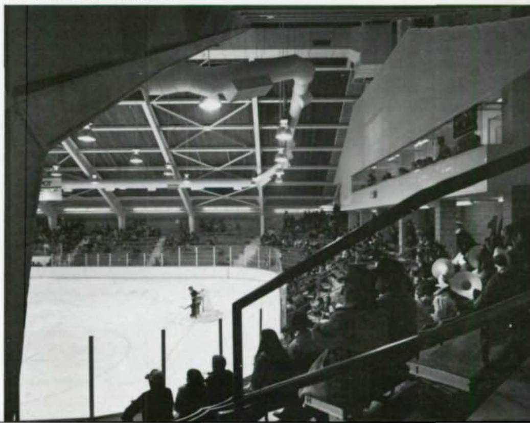
Remodelled Alexander H. Bright Hockey Center, clear-spanned with steel bents, was updated to include new ice arena, boards and seating for 2,800. Photos by Sam Sweezy (above) and Nick Wheeler (below).
