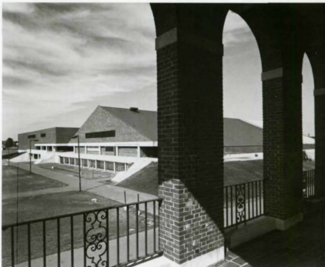
Remodelled Alexander H. Bright Hockey Center, clear-spanned with steel bents, was updated to include new ice arena, boards and seating for 2,800. Photos by Sam Sweezy (above) and Nick Wheeler (below).
