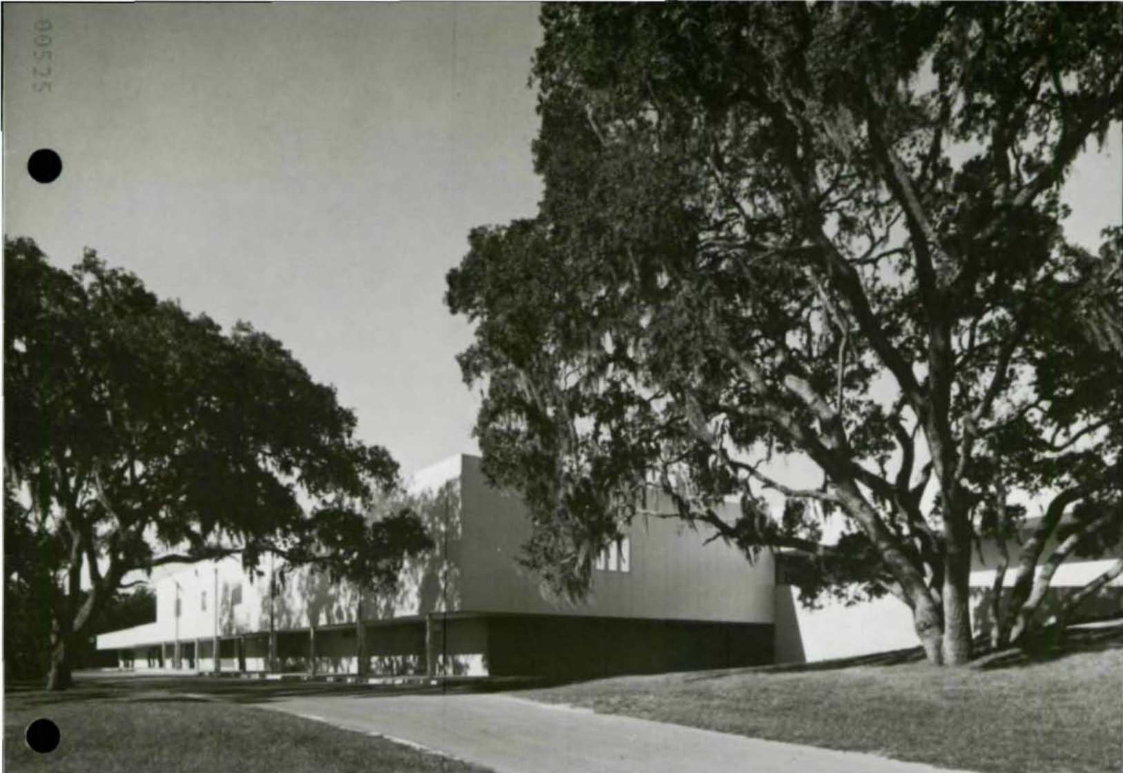
Ridgewood Junior High—a compact, open-planned structure for 1,500 students. New Port Richey, Florida.
